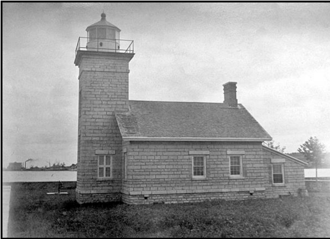
ABOVE, 1885 view showing original configuration; BELOW, 1903, after extension of tower and introduction of new frame extension
