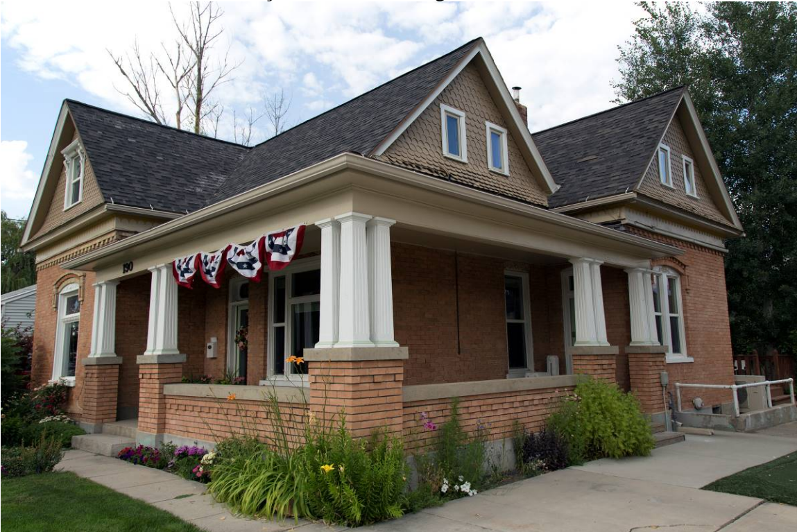
2 of 15. View of southwest façade. Camera facing northeast.
