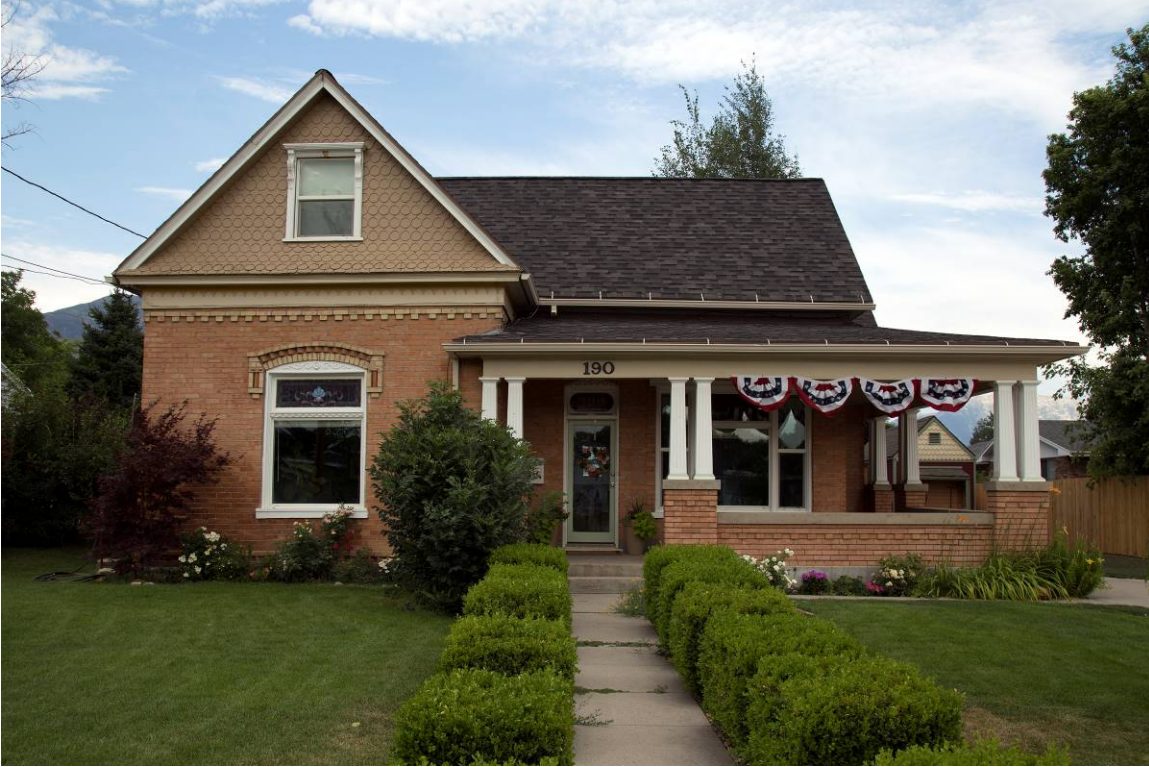
1 of 15. View of west (front) façade. Camera facing east.
