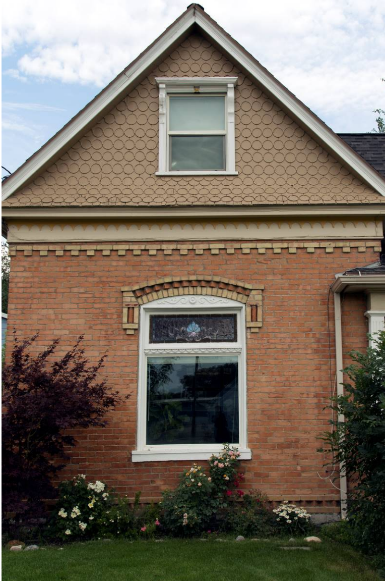
10 of 15. Projecting wing detail. Camera facing east.
