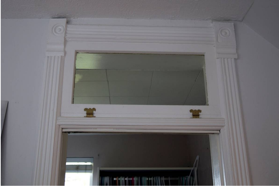
13 of 15. Transom window and casing/trim detail. Camera facing south.
