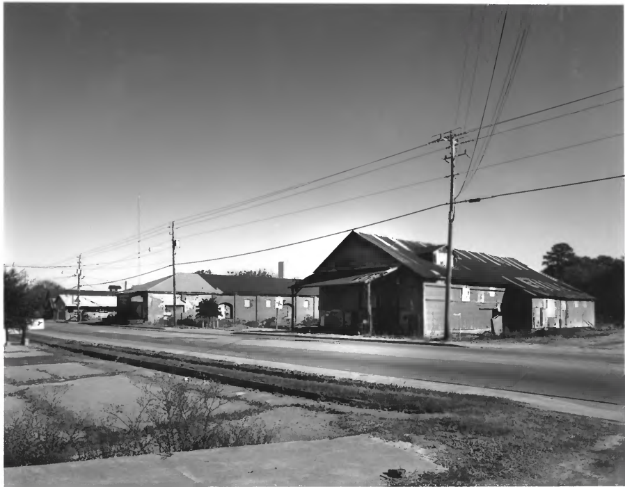
SANDERSVILLE COMMERCIAL AND INDUSTRIAL HISTORIC DISTRICT SANDERSVILLE, WASHINGTON COUNTY, GEORGIA PHOTOGRAPH 34 OF 35
