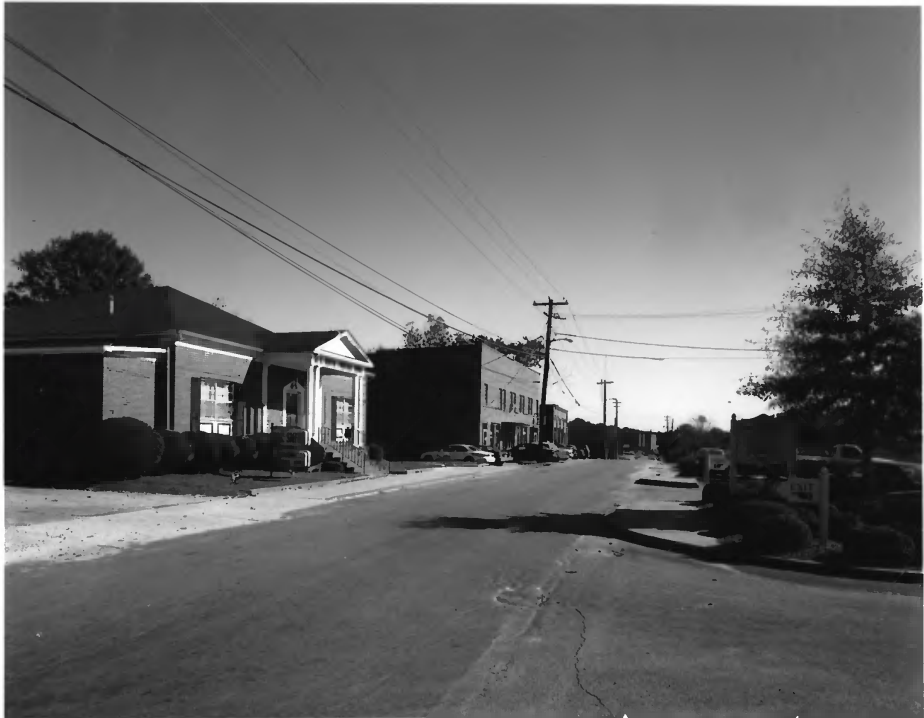
SANDERSVILLE COMMERCIAL AND INDUSTRIAL HISTORIC DISTRICT SANDERSVILLE, WASHINGTON COUNTY, GEORGIA PHOTOGRAPH 19 OF 36
