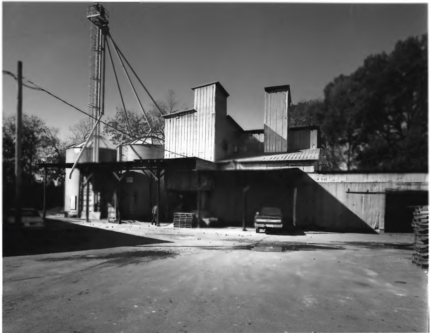
SANDERSVILLE COMMERCIAL AND INDUSTRIAL HISTORIC DISTRICT SANDERSVILLE, WASHINGTON COUNTY, GEORGIA PHOTOGRAPH 28 OF 35
