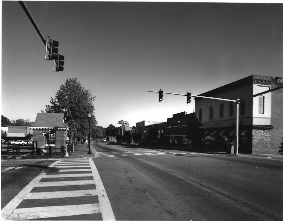
SANDERSVILLE COMMERCIAL AND INDUSTRIAL HISTORIC DISTRICT SANDERSVILLE, WASHINGTON COUNTY, GEORGIA PHOTOGRAPH 14 OF 35
