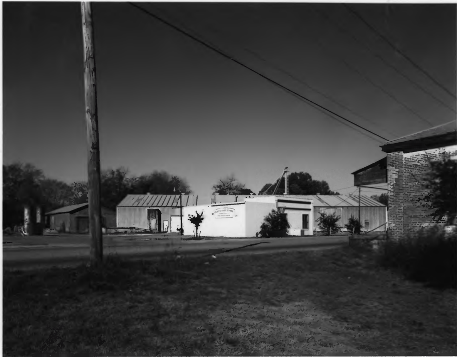
SANDERSVILLE COMMERCIAL AND INDUSTRIAL HISTORIC DISTRICT SANDERSVILLE, WASHINGTON COUNTY, GEORGIA PHOTOGRAPH 25 OF 35
