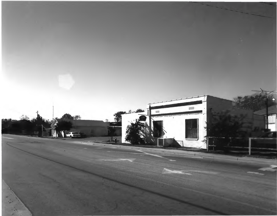
SANDERSVILLE COMMERCIAL AND INDUSTRIAL HISTORIC DISTRICT SANDERSVILLE, WASHINGTON COUNTY, GEORGIA PHOTOGRAPH 24 OF 35
