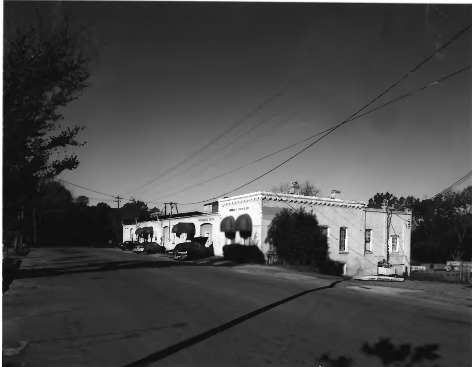
SANDERSVILLE COMMERCIAL AND INDUSTRIAL HISTORIC DISTRICT SANDERSVILLE, WASHINGTON COUNTY, GEORGIA PHOTOGRAPH 5 OF 35
