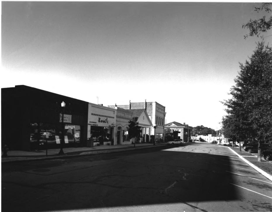
SANDERSVILLE COMMERCIAL AND INDUSTRIAL HISTORIC DISTRICT SANDERSVILLE, WASHINGTON COUNTY, GEORGIA PHOTOGRAPH 6 of 35
