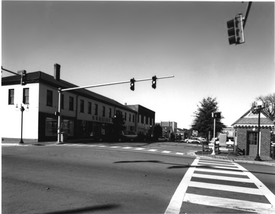
SANDERSVILLE COMMERCIAL AND INDUSTRIAL HISTORIC DISTRICT SANDERSVILLE, WASHINGTON COUNTY, GEORGIA PHOTOGRAPH 7 OF 35
