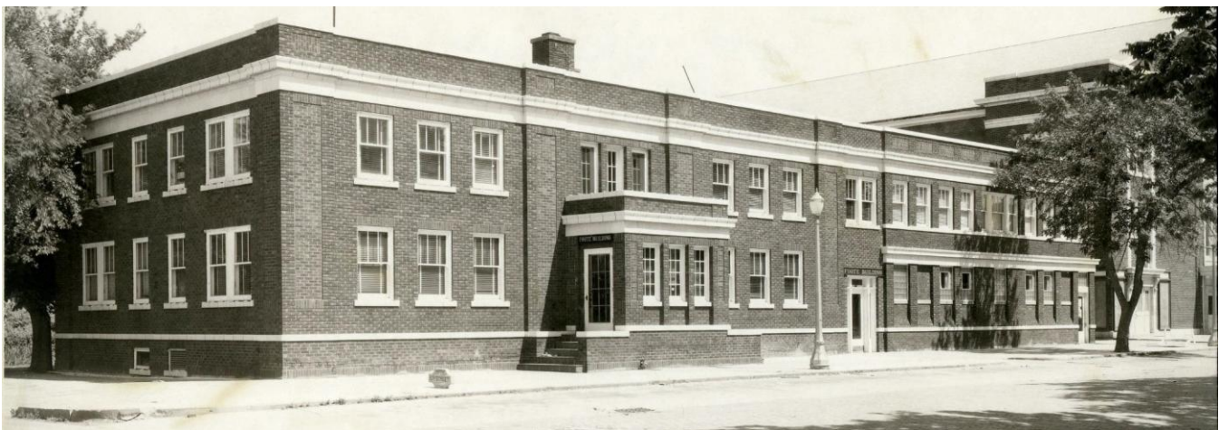
Figure 6: Front façade of the Foote Clinic building, c. 1950s. The 1928 building features the new ground level façade of alternating pilasters and glass block windows. The 1924 Clinic building retains its historic entryway. (Adams County Historical Society)
