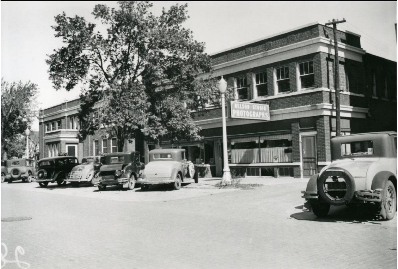
Figure 5: Foote Clinic Buildings, c. 1932-1935. The 1928 building retains its original storefront in this photograph. The current ground-level façade most likely dates to the 1940 or 1944 renovations of the Foote Clinic. (Adams County Historical Society)
