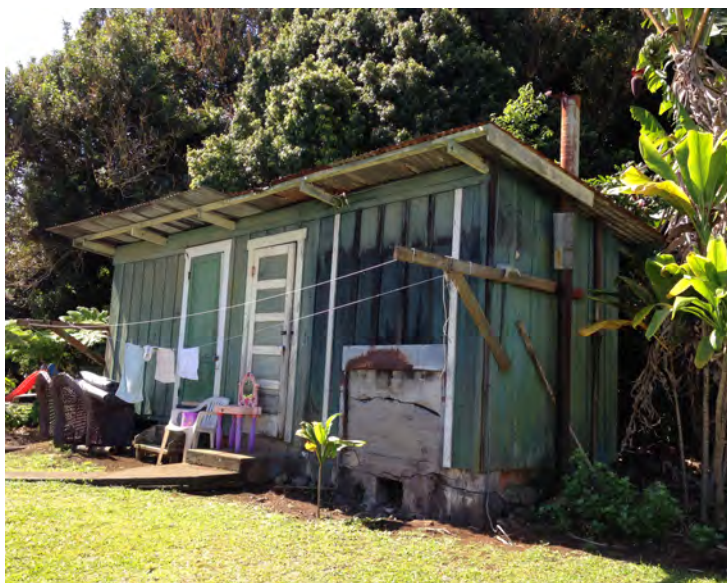
Left: the Tofukuji Hospital Laundry/ Furo Building shows two sections of the same building with different board-and-batten construction. The exhaust chimney is in the upper right of the photo. Right: an exterior detail view of the concrete furo fire chamber.
