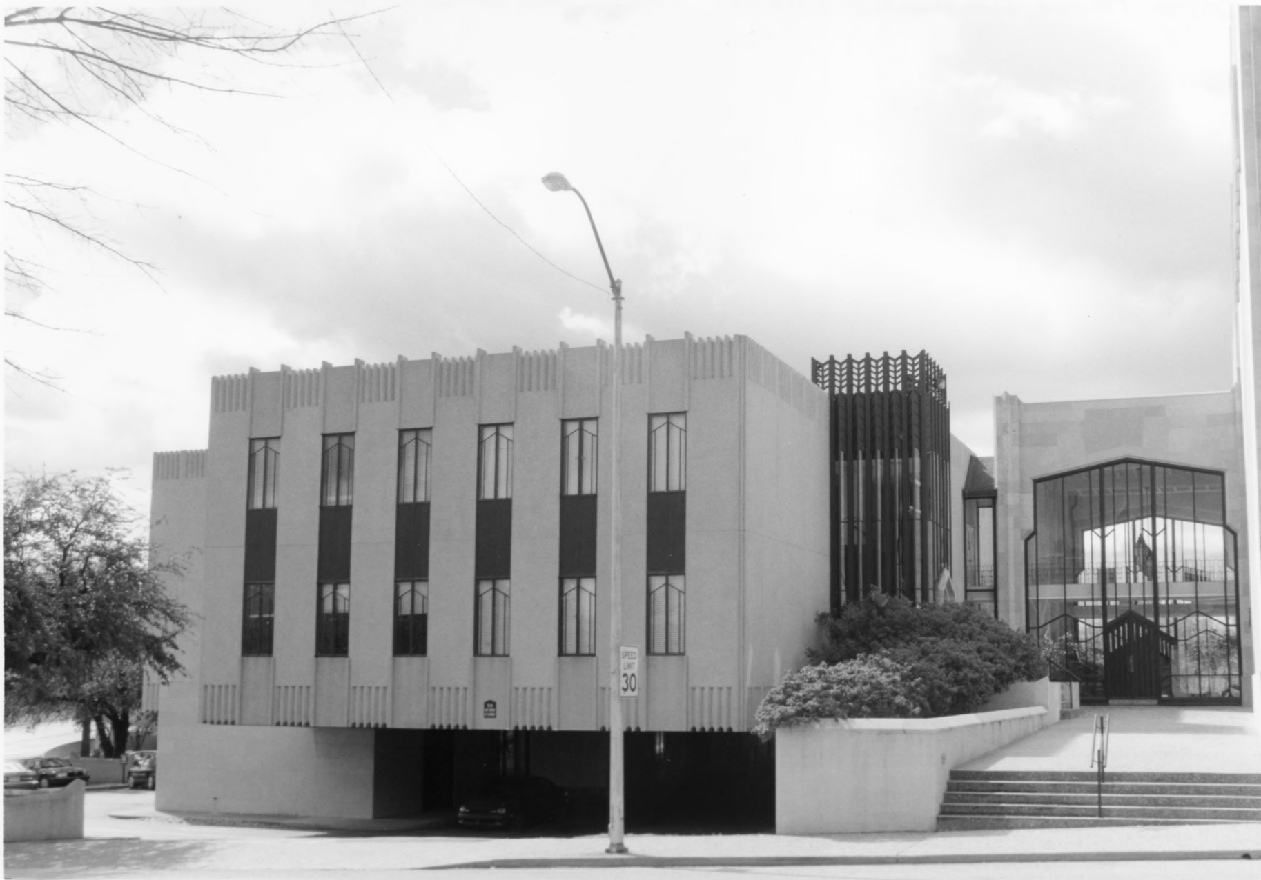
Photo #3 Boston Avenue Methodist Episcopal Church, Tulsa, Oklahoma North side, education wing and porte cochere
