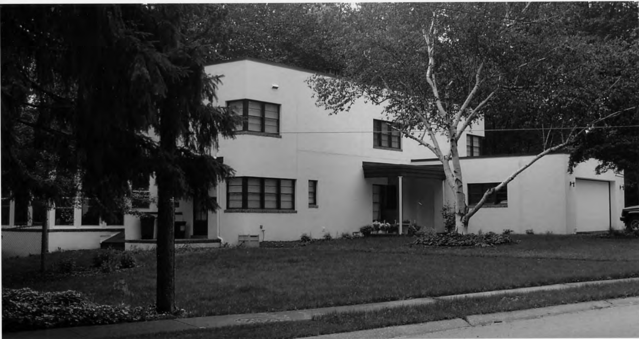
Carswell House_New Castle County_DE facade view from Briar Lane
