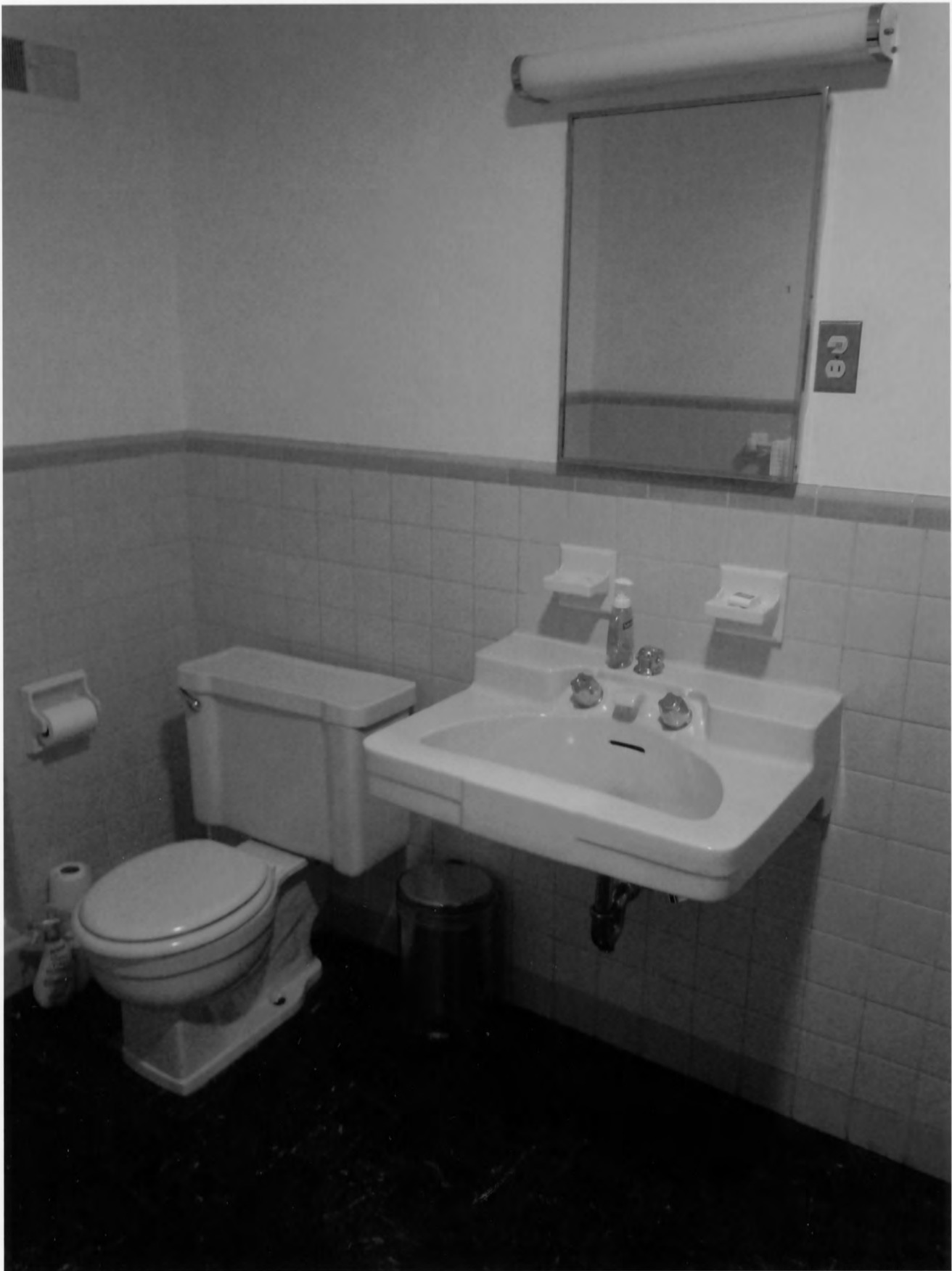
Carswell House, New Castle County, DE Master bedroom - original ceramic tiles and plumbing fixtures - Crane Drexel series designed Henry Dreyfuss 18 of 25
