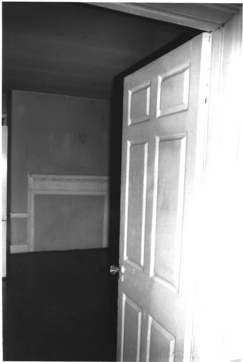
PHOTO # 6 OF 6 NJ BURLINGTON Co. ISAAC COLLINS HOUSE
