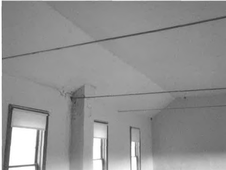
Tie rods and cove ceiling of church interior, View to the East
