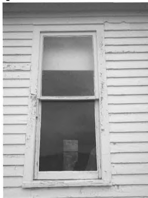
Details of exterior windows (rose wheel window in tower to left and 1/1 double-hung on main building to right)
