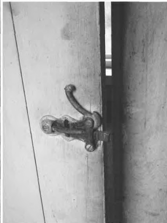
Detail of closet interior showing beaded board ceiling and walls (left) and closet door hardware (to right)
