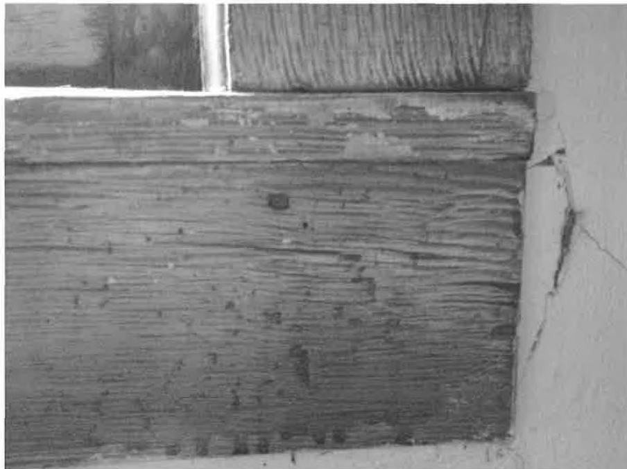
Details of painted wood graining on interior woodwork of church (baseboard upper left; door surround upper right; and window surround below)
