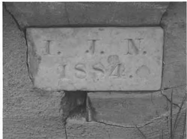
Details of foundation (parged brick foundation to left and inscribed marble cornerstone to right)
