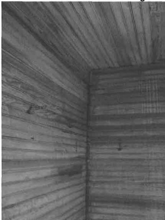
Detail of closet interior showing beaded board ceiling and walls (left) and closet door hardware (to right)
