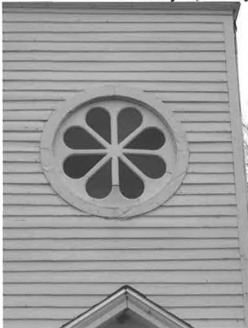
Details of exterior windows (rose wheel window in tower to left and 1/1 double-hung on main building to right)
