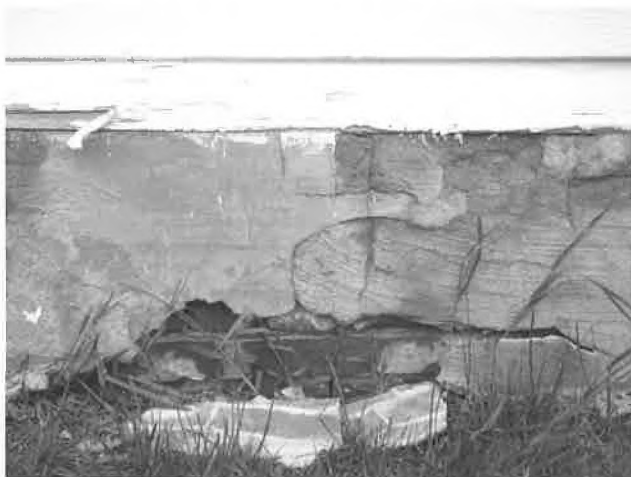
Details of foundation (parged brick foundation to left and inscribed marble cornerstone to right)
