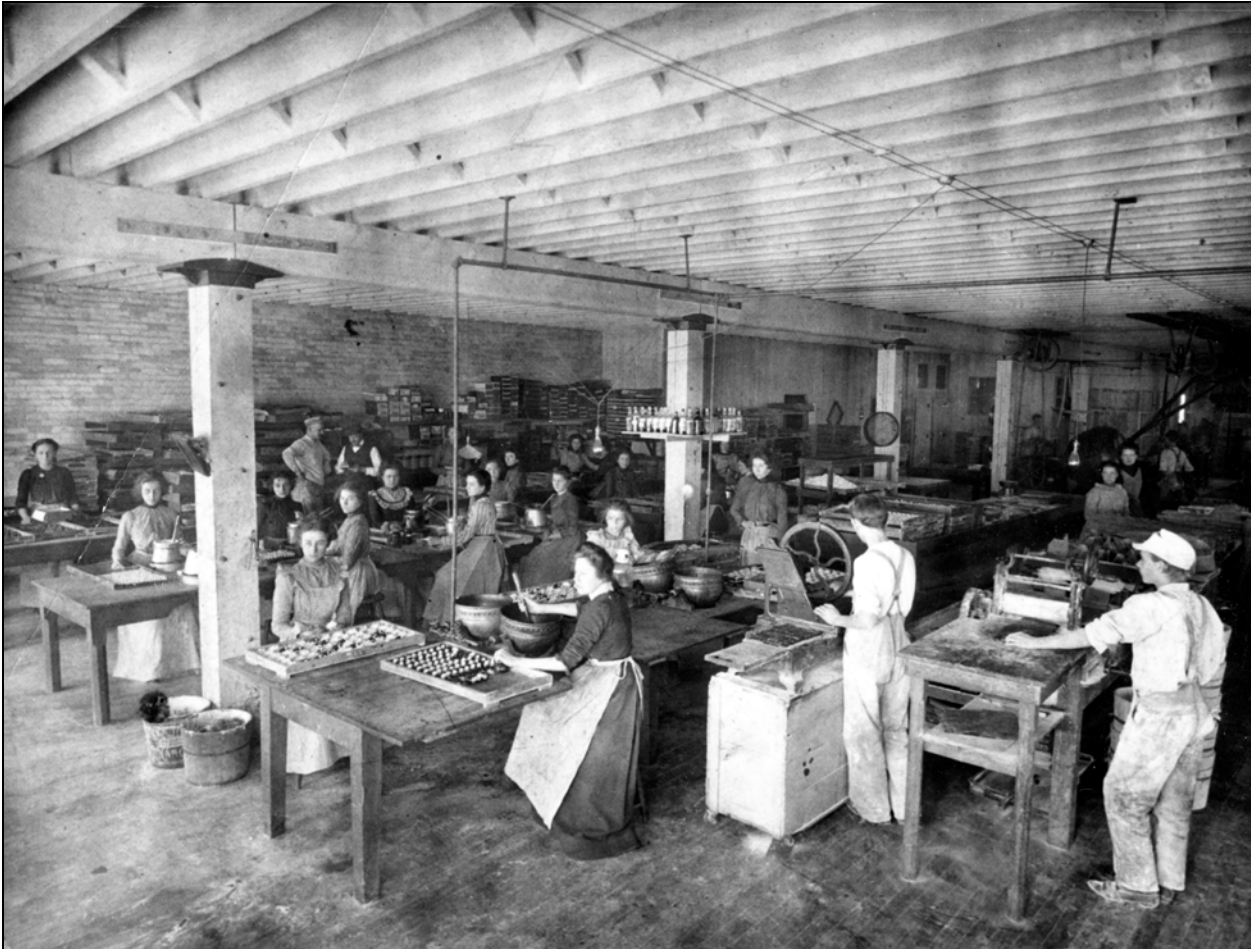
Historic Photograph #6: Joseph B. Funke Company, third floor, circa 1900 photograph.
