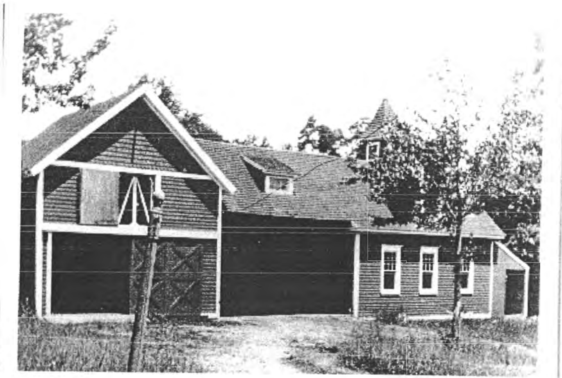
Figure 12. Carriage House/Stable, northeast view, early 20th century. Taken before the construction of the rear addition, the photo documents that the west end was used for vehicular storage and that the central bay was originally open. (Portland Place Collection, MCPS)
