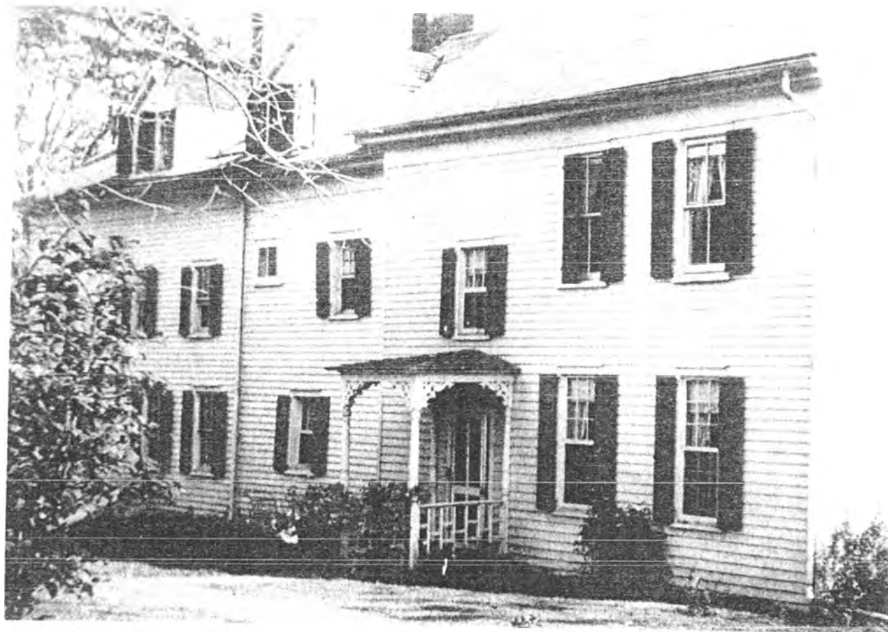
Figure 4. House, SE view, late 19th/early 20th century before west addition was constructed. The entry porch & 2/2 sash windows date to the “country place” renovations, as does the east addition left of the downspout. (Portland Place Collection, MCPS)
