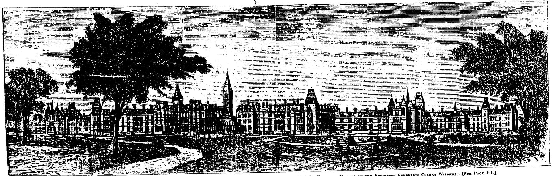
HUDSON RIVER STATE HOSPITAL FOR THE INSANE, POUGHKEEPSIE, DUTCHESS COUNTY, NEW YORK.—FROM THE DESIGNS OF THE ARCHITECT, FREDERICK CLARKE WITMERS.—[SEE PAGE 191.]
