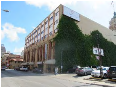
ID# 38 Riverwalk Plaza Hotel Main Plaza/ 100 Villita Street 1926/ ca. 1968 Non-Contributing
