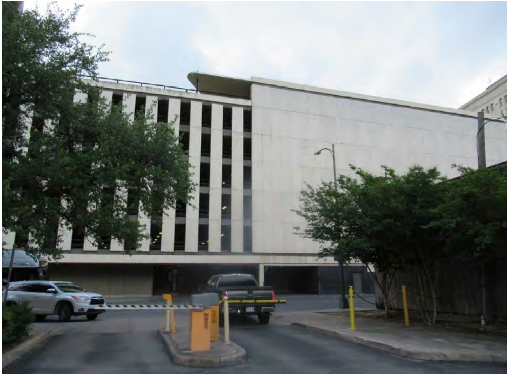
Photo #17: Frost Bank Parking Garage, 109 N. Main, 117 W. Commerce Street, West façade, camera facing east
