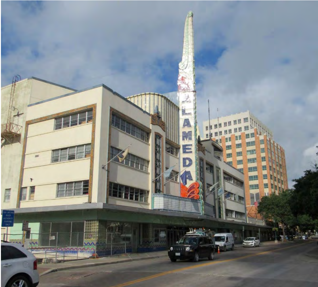
Photo #22: Alameda Theater, 303-314 W. Houston Street, Northeast oblique, camera facing southwest
