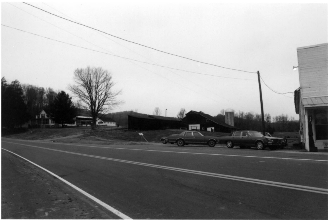
Forbus Historic District Fentress County TN
