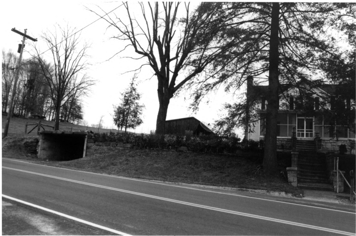
Forbus Historic District Fentress County TN
