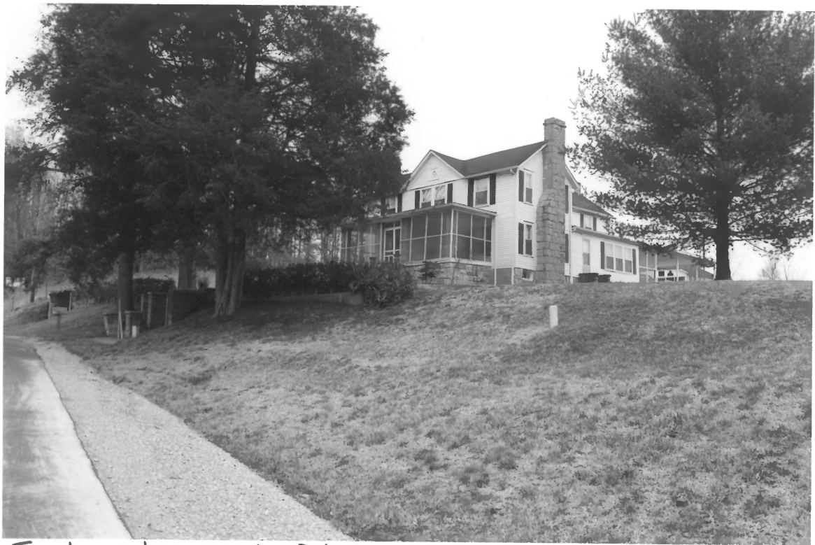
Forbus Historic District Fentress County TN
