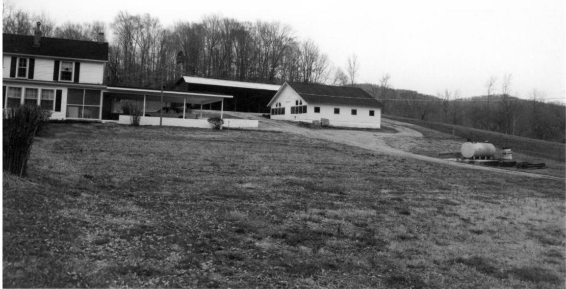
Forbus Historic District Fentress County TN
