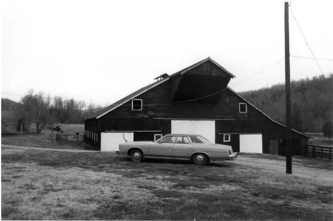
Forbus Historic District Fentress County TN
