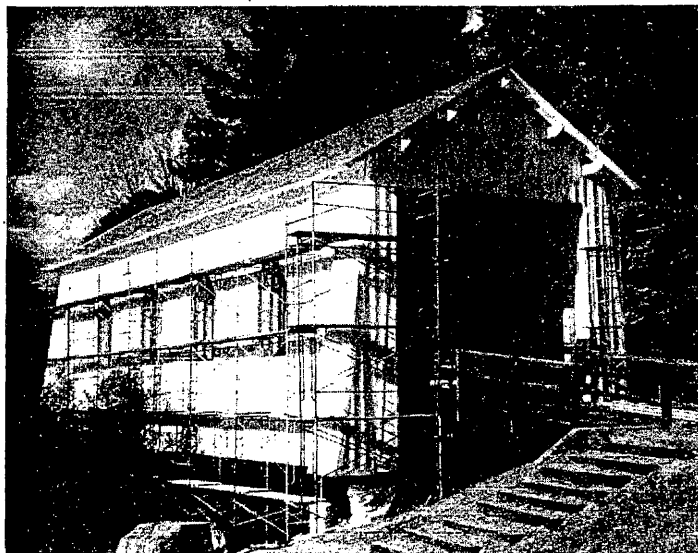
Lower photo: Ritner Creek Bridge in Polk County now fully refurbished. This view shows the scaffolding used to replace the roof and apply a new coat of white paint. Also note the steps on the right end of the photo which allow visitors a safer walk to the water's edge.
