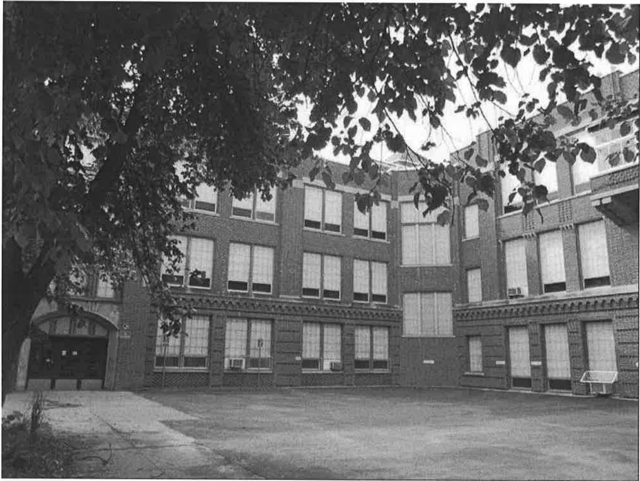
PHOTO 0005: EAST AND SOUTH ELVATIONS OF "T" (Greenhouse in top right corner)—VIEW TO THE NORTHWEST
