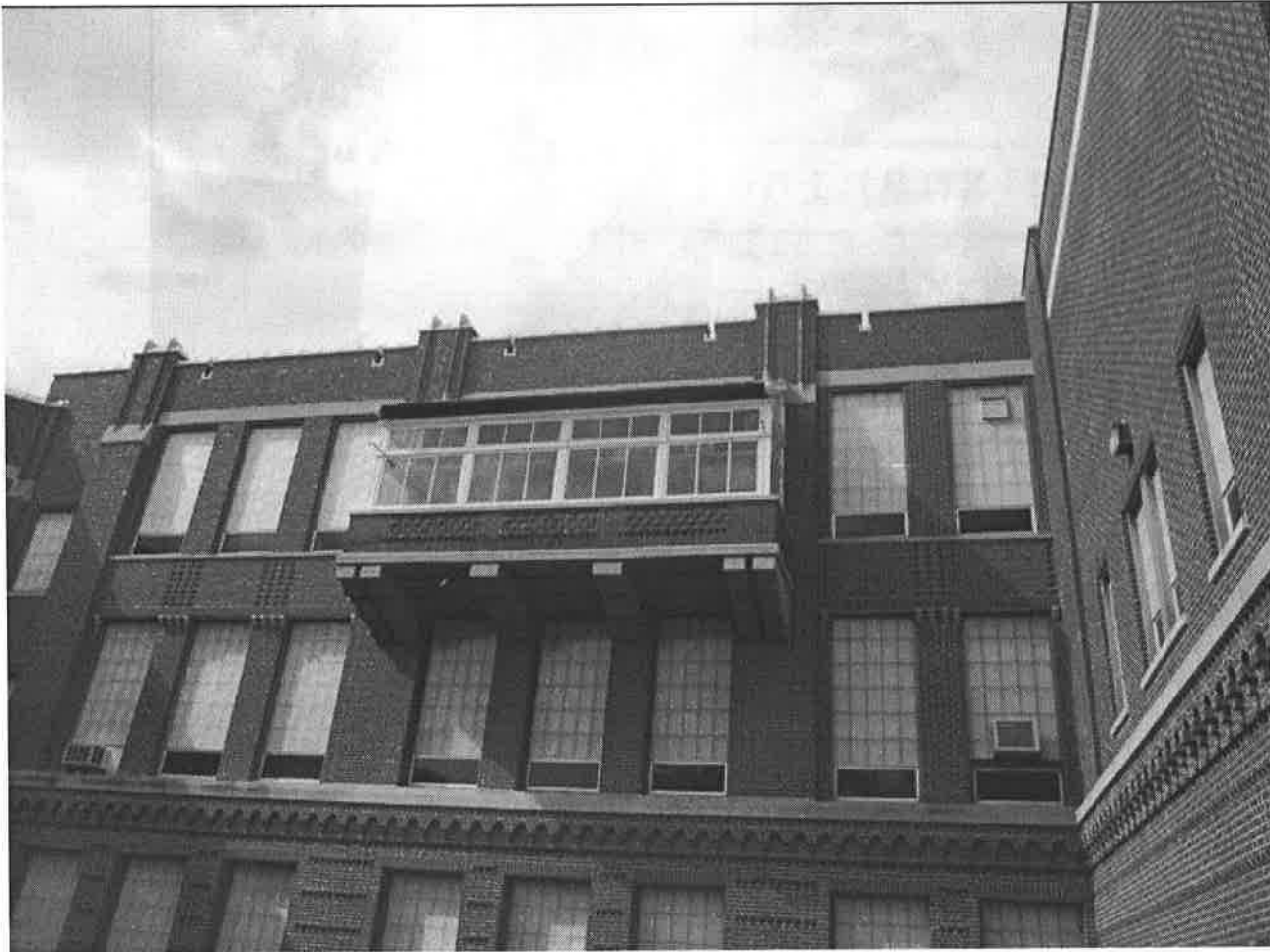
PHOTO 0006: SOUTH GREENHOUSE ELEVATION-VIEW TO THE NORTH
