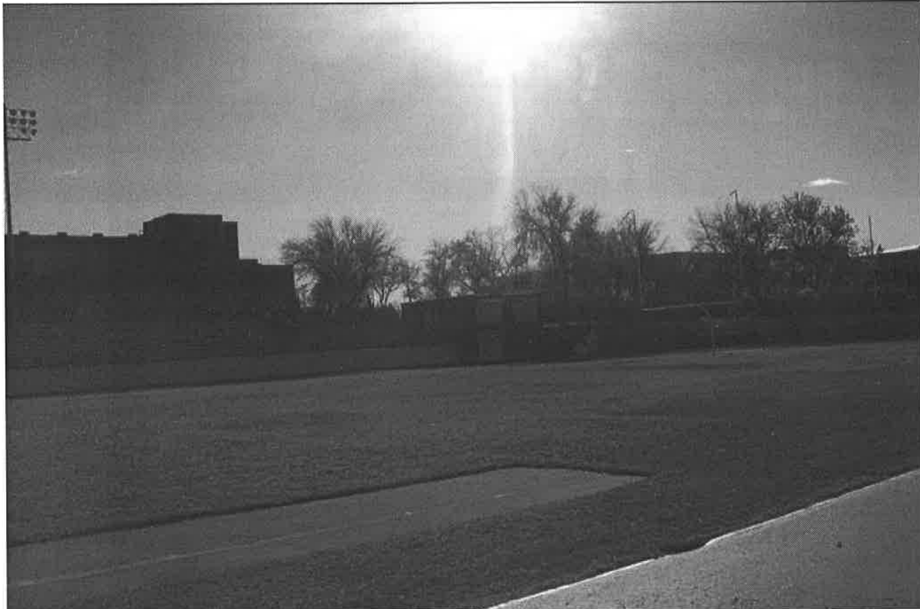
PHOTO 0016: EAST BLEACHER, FIELD, and SOUTH FLANKING BUILDING—VIEW TO THE SOUTHEAST
