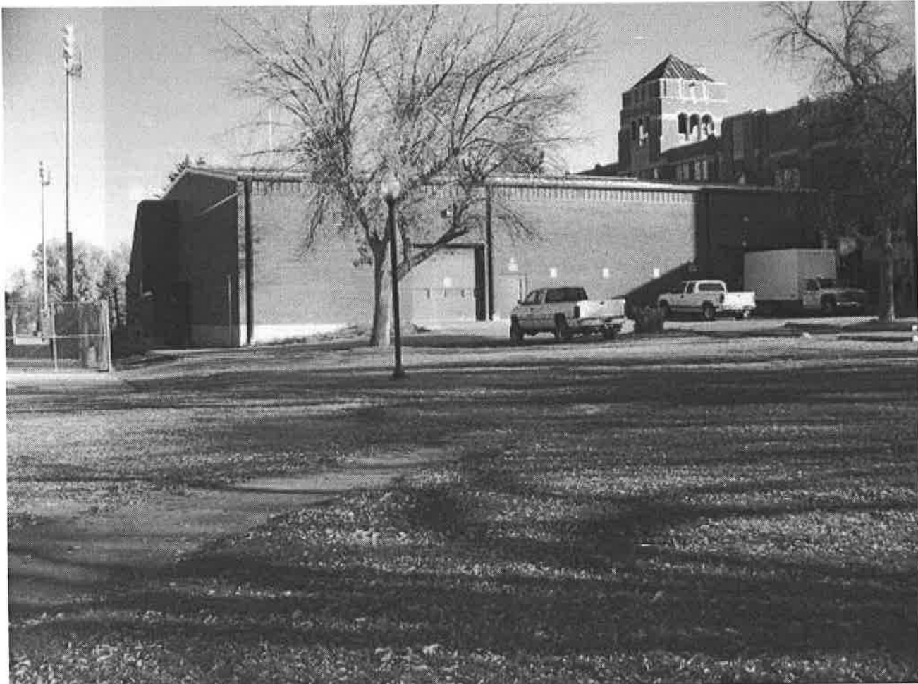
PHOTO 0018: INDUSTRIAL ARTS BUILDING, WEST and SOUTH ELEVATIONS—VIEW TO THE NORTHEAST
