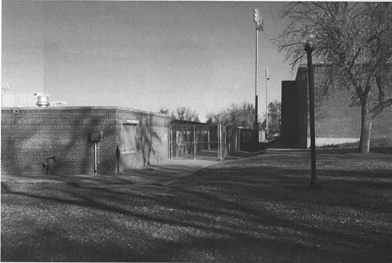
PHOTO 0015: FLANKING BUILDING OF EAST BLEACHER, SOUTH AND EAST ELEVATIONS (Industrial Arts Building to Right)—VIEW TO THE NORTH-NORTHWEST
