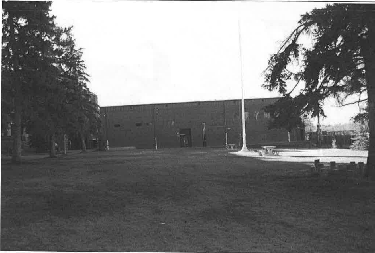
PHOTO 0019: INDUSTRIAL ARTS BUILDING, NORTH ELEVATION—VIEW TO THE SOUTH
