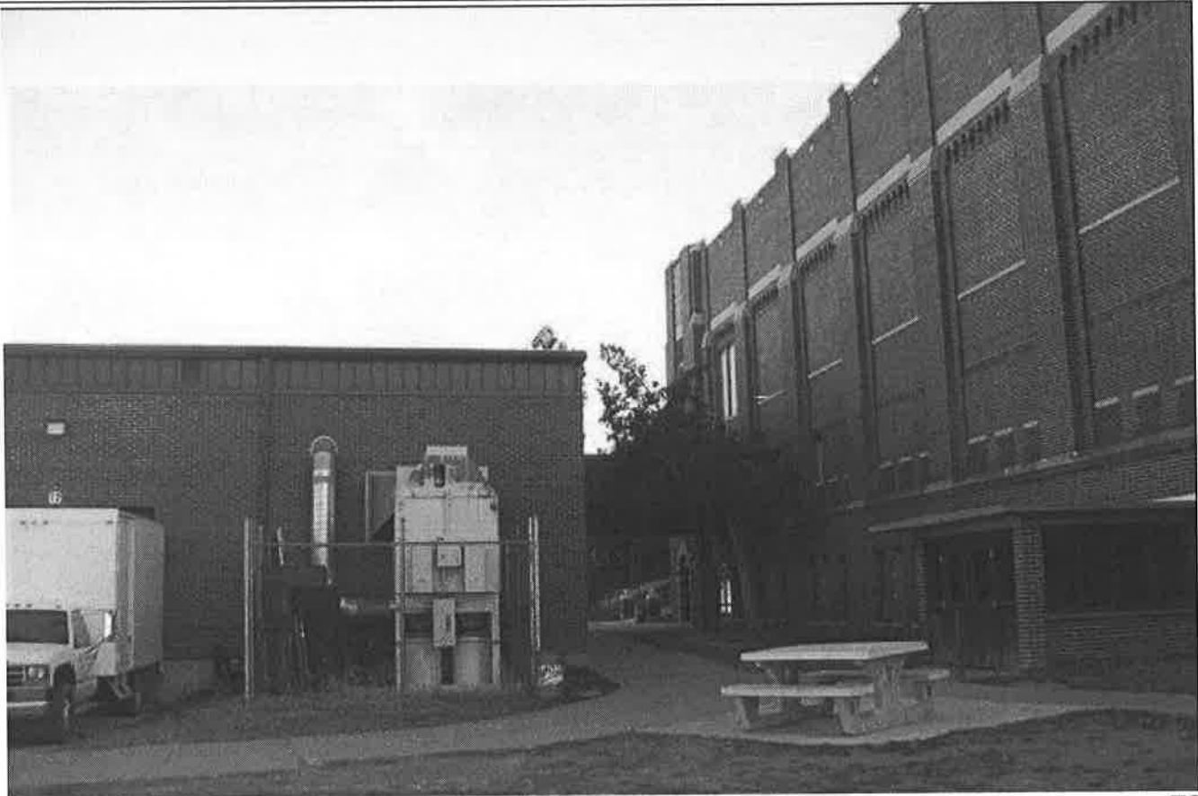
PHOTO 0008: WEST THEATRE ELEVATION AND SOUTH INDUSTRIAL ARTS BUILDING ELEVATION-VIEW TO THE NORTH
