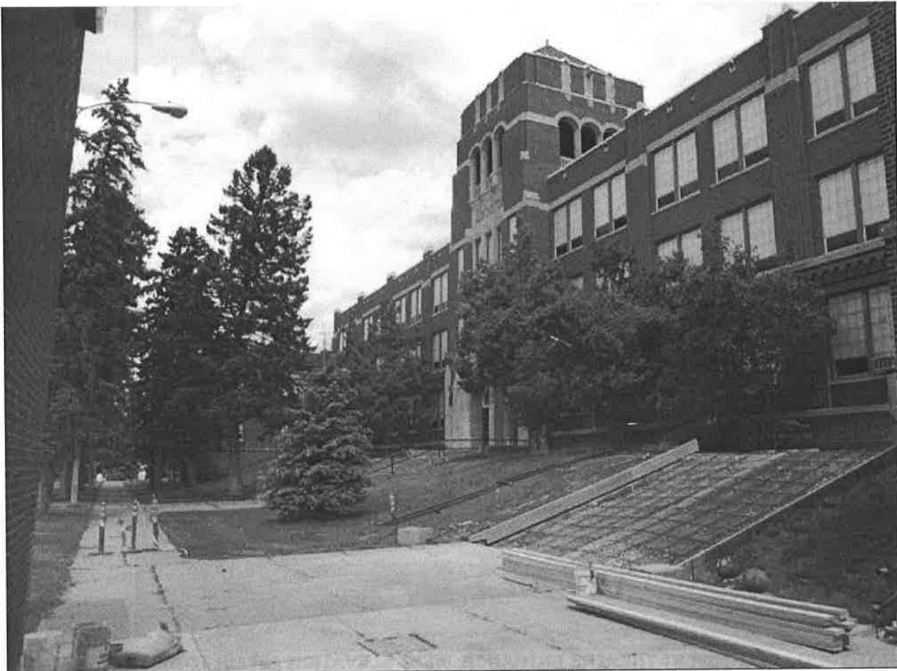
PHOTO 0002: WEST ELEVATION-VIEW TO THE NORTHEAST
