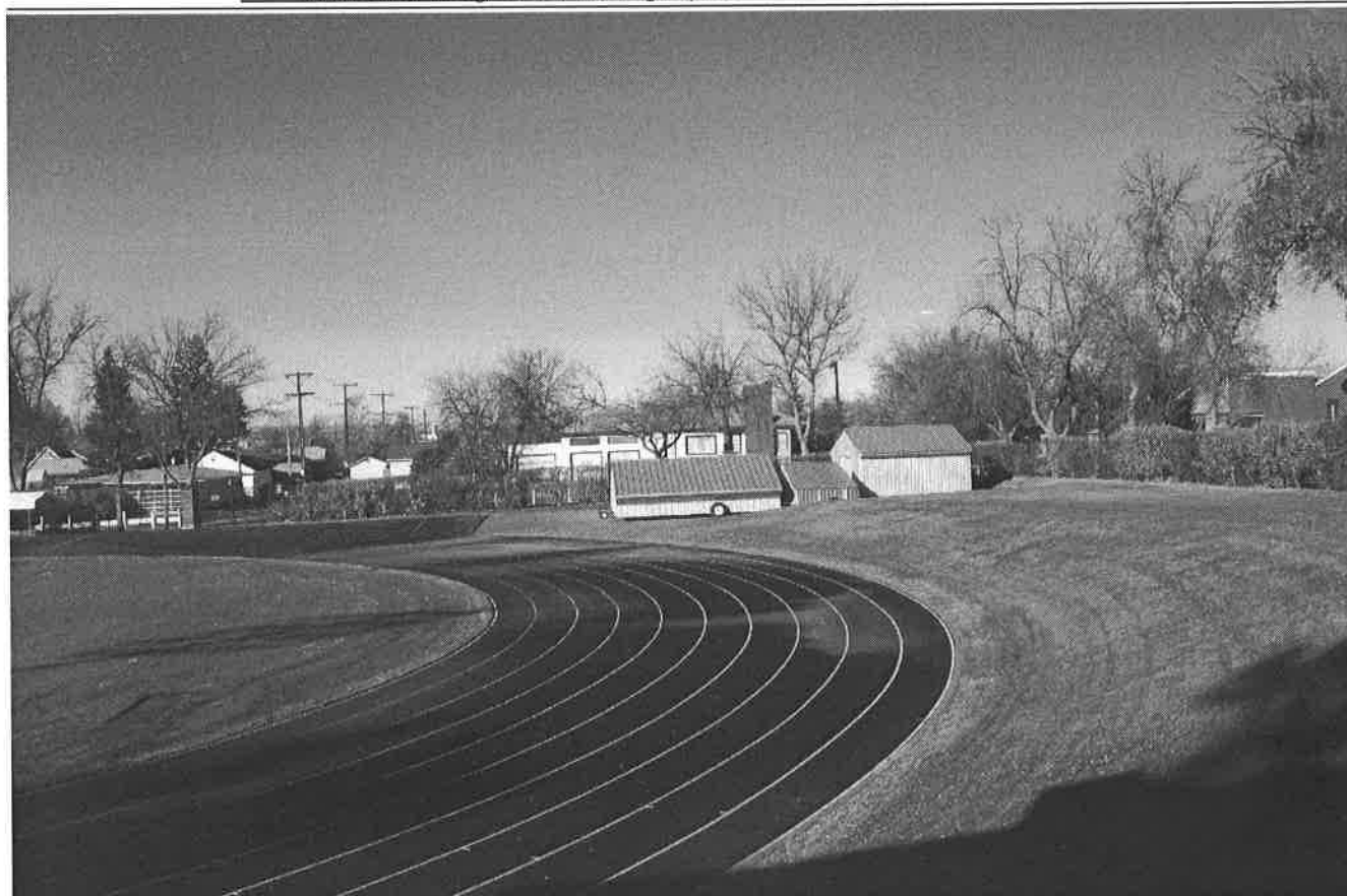
PHOTO 0022: OVERVIEW OF NONPERMANENT MAINTENANCE BUILDINGS (TWO) and PERMANENT MAINTENANCE BUILDING (ONE) [NORTH OF WEST BLEACHERS] WITH TRACK IN FOREGROUND, EAST ELEVATIONS—VIEW TO THE WEST
