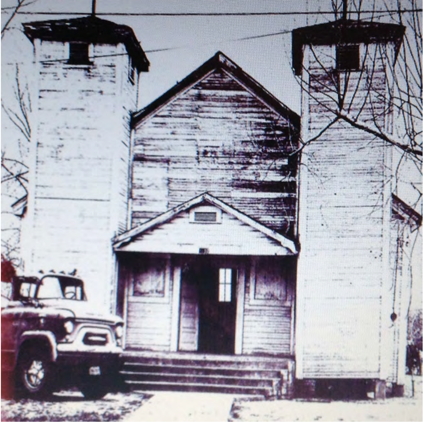
Figure 8. Greater Ebenezer Baptist Church, where many of the BCVL and Deacons meetings, as well as other civil rights meetings, were held. This was the only church that allowed civil rights meetings to occur there in Bogalusa. The church was renovated and updated and no longer looks like this today, but is still used by the community and was recently added to the Louisiana African American Heritage Trail. Image courtesy of Rev. Dr. Raymond Mims.
