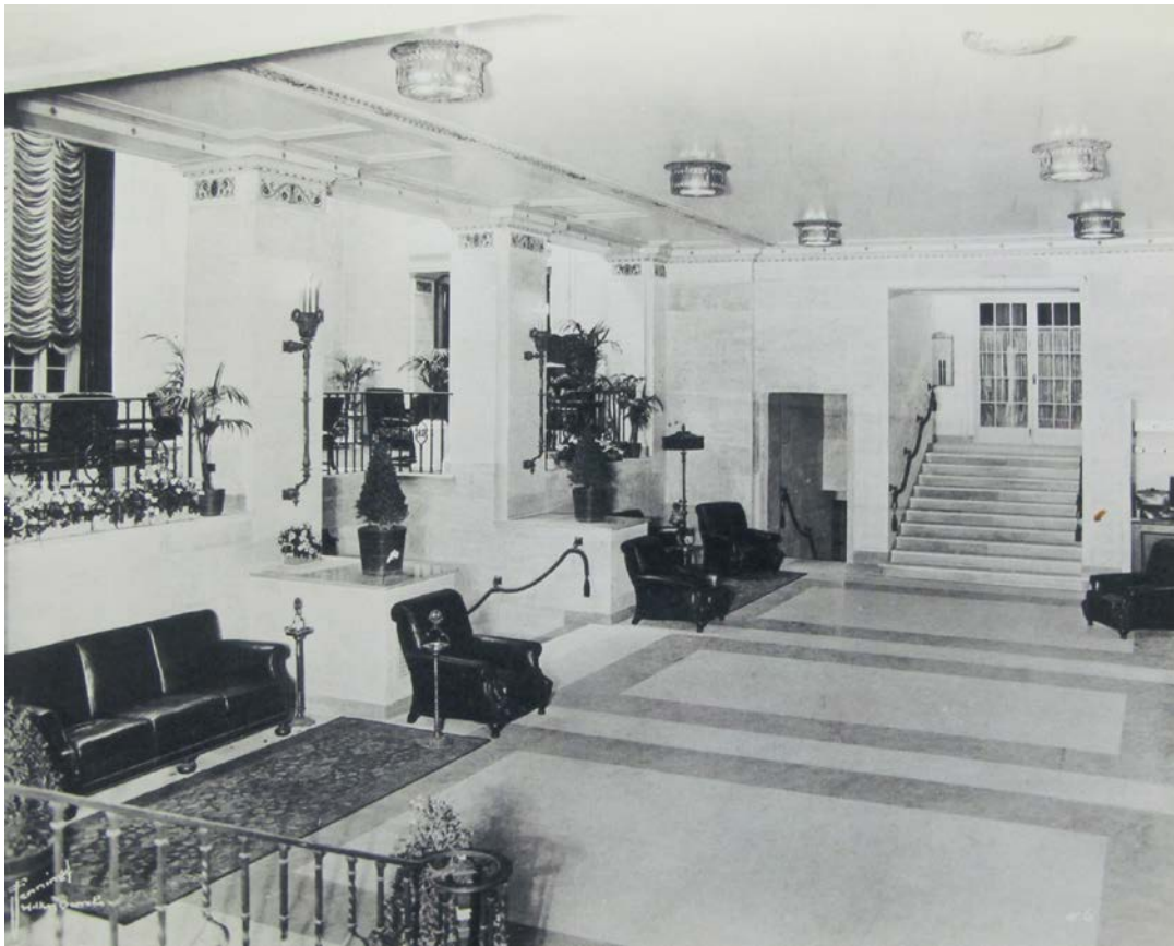
Figure 8 – Lobby, looking north, 1924.
