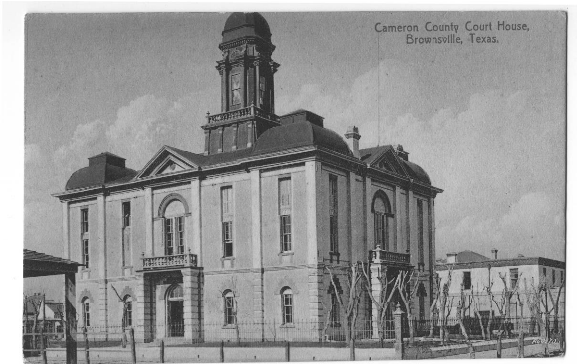
Figure 11: Circa 1907 View of South Elevation of 1883 Cameron County Courthouse and Cameron County Jail. The rear wall of the jail yard is visible at lower right. This confirms the character defining buttresses were part of the original 1883 design. Photo courtesy THC.
