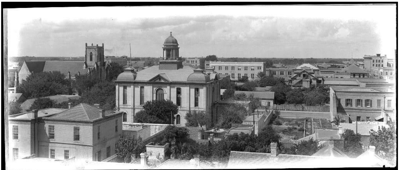
Figure 12: View of Rear (North) Elevation of 1883 Cameron County Courthouse with County Jail in Foreground. Photo courtesy of THC.
