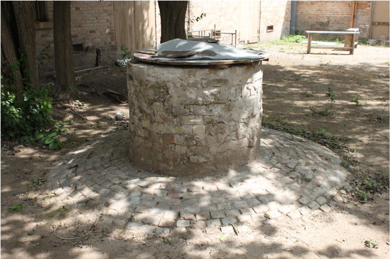
Cistern in patio, camera facing east.
