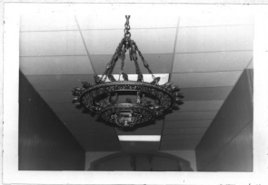
INTERIOR DETAIL - LIGHT FIXTURE
