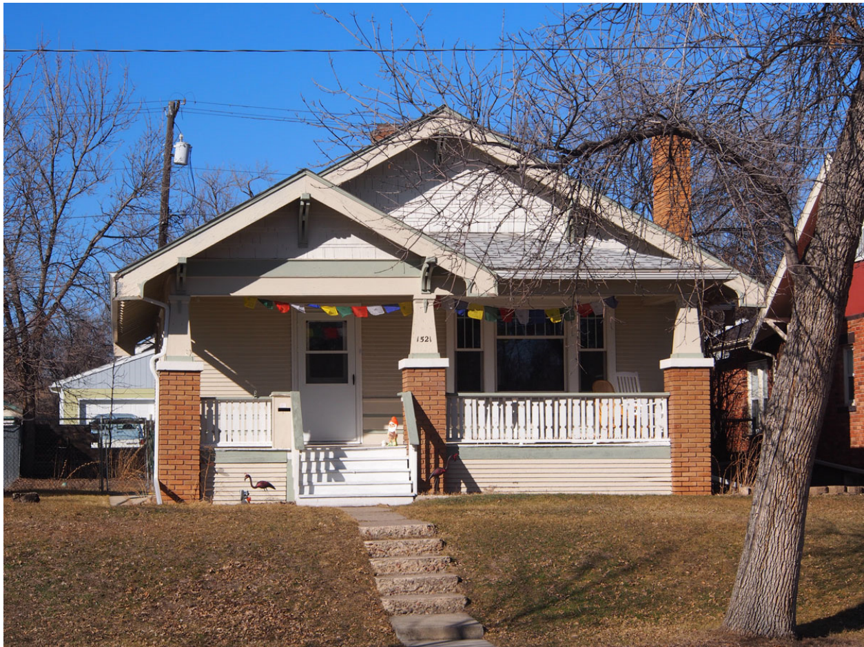
Description of Photograph: Emma Barkenmeyer House, 1521 Central, view to north. Photo No. MT_CascadeCounty_EastSideNeighborhoodHistoricDistrict_0008
