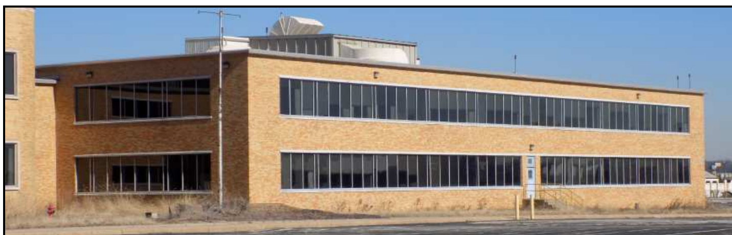
Figure 16: Portion F, ancillary building containing the engineering department annex before 1945. Top is south elevation; bottom is north. Source: Photographs by Matt Bivens, 2016.
