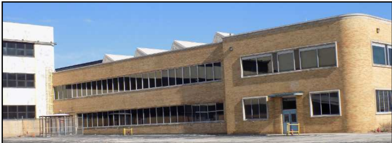
Figure 6: West elevation of portion A (right side) showing projecting front and skylights. The south-facing elevation of portion C (AKA High Bay) is at left. Source, Matt Bivens photograph, January 2016.
