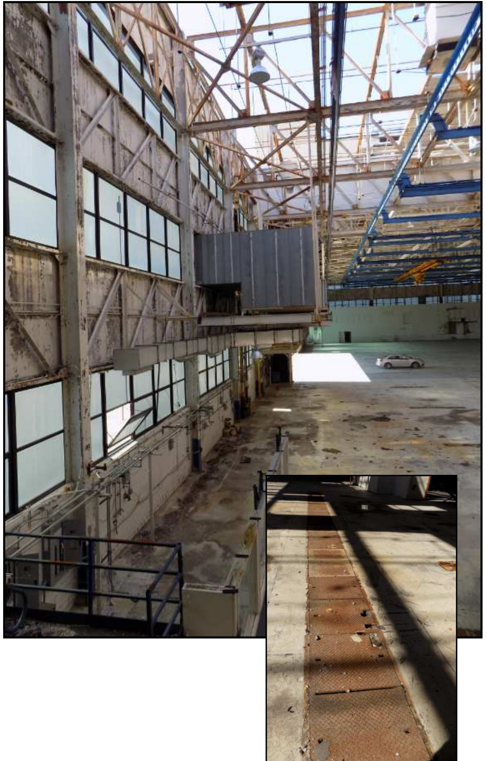
Figure 21A (large pic) and 21B (small pic): Portion C, interior of High Bay area (21A) and assembly line tracks (21B). Source: Matt Bivens, photograph 1-2016.
