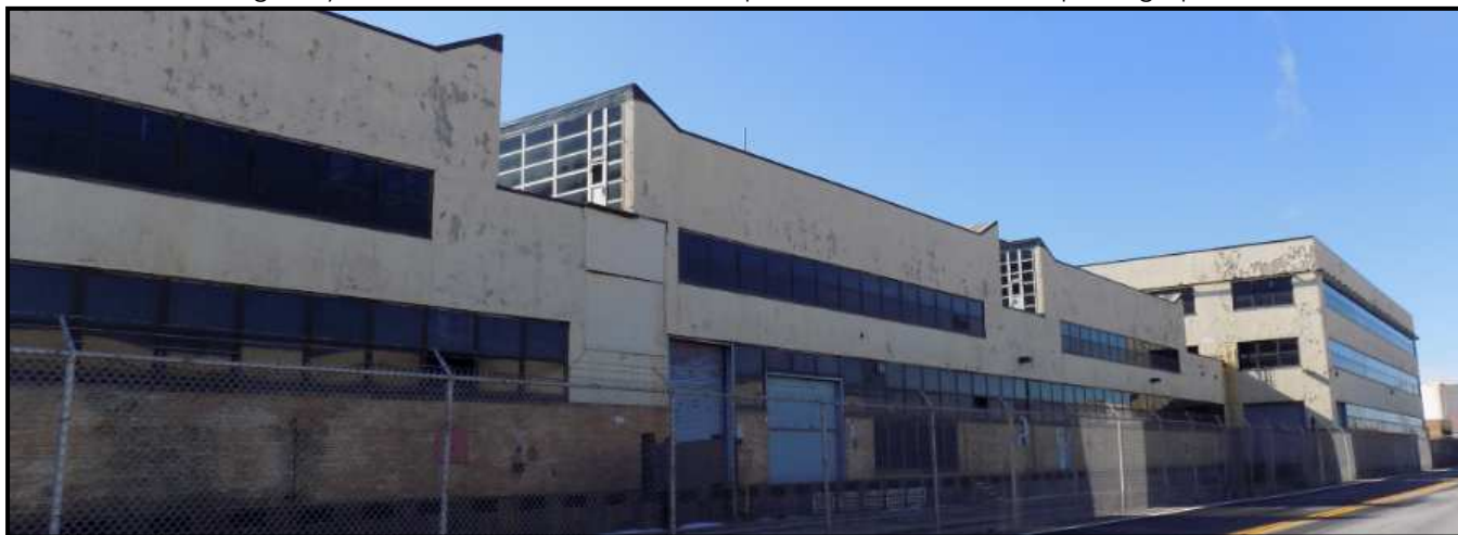
Figure 10: North elevation of factory with High Bay (C-right) & Low Bay (B-left); the Low Bay is set back from the street and High Bay to accommodate the railroad spur. Source, Matt Bivens photograph, 1-2016.
