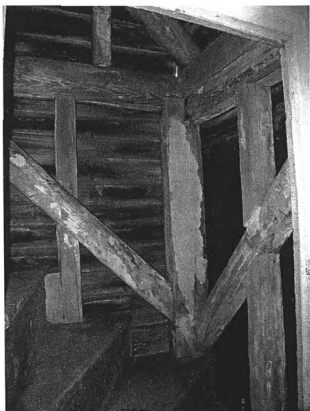
Figure 8: timber framing of second floor
