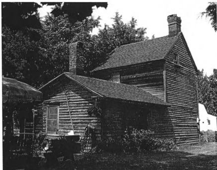
Figure 10: the house before restoration, 2002
