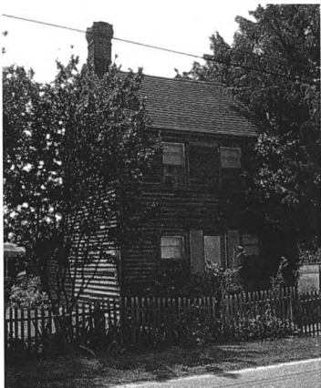
Figure 9: the house before restoration, 2002
