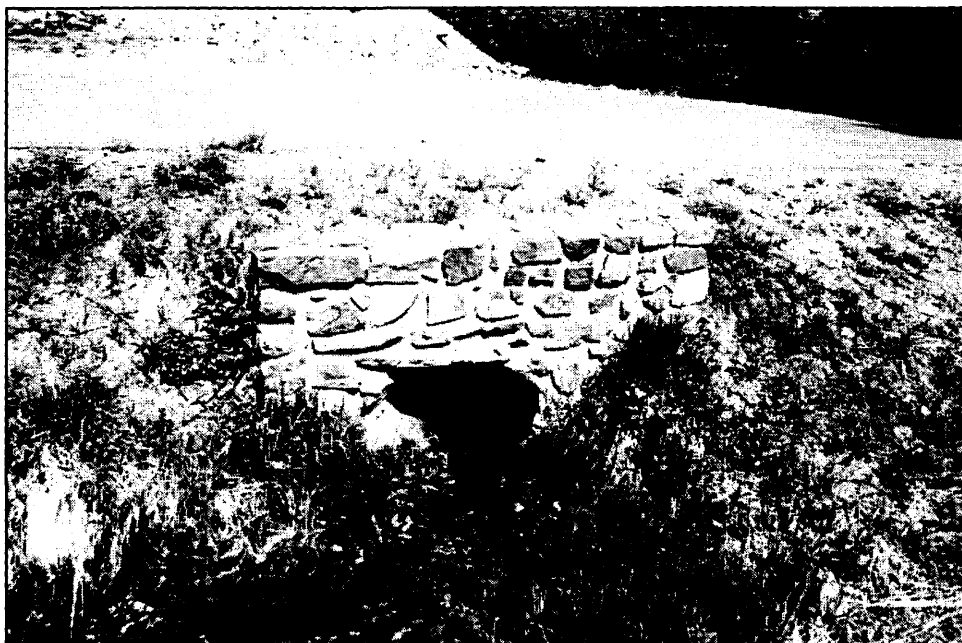
Photo 12: Stone Headwall on concrete culvert – on West Sulphur Creek, view to east.
