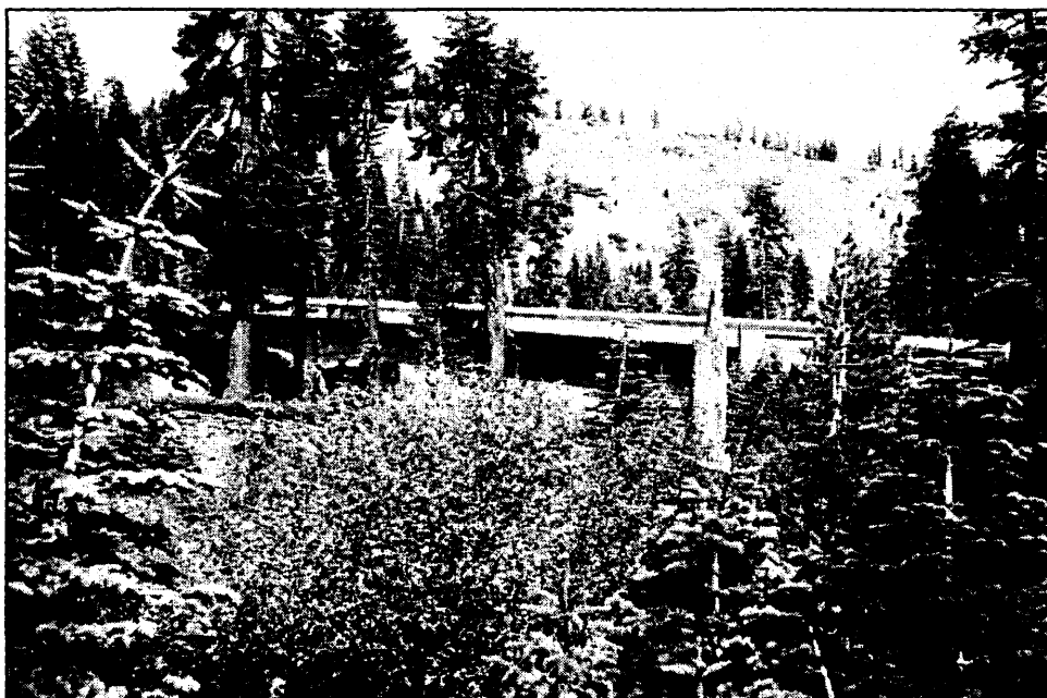
Photo 13: Bridge over West Sulphur Creek, view to east.
