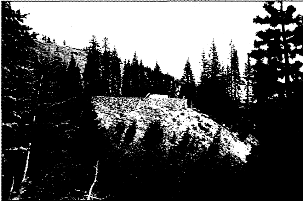
Photo 10: Guardrail near bridge project – Sulphur Works, view to east.
