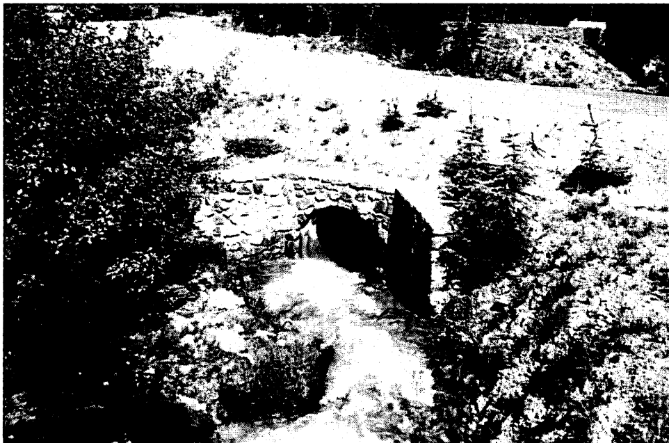
Photo 11: Stone Headwall on concrete culvert – on West Sulphur Creek, view to SE.
