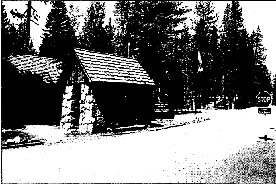
Photo 2: Northwest Entrance Station – Entrance Kiosk and residence, view to west.
