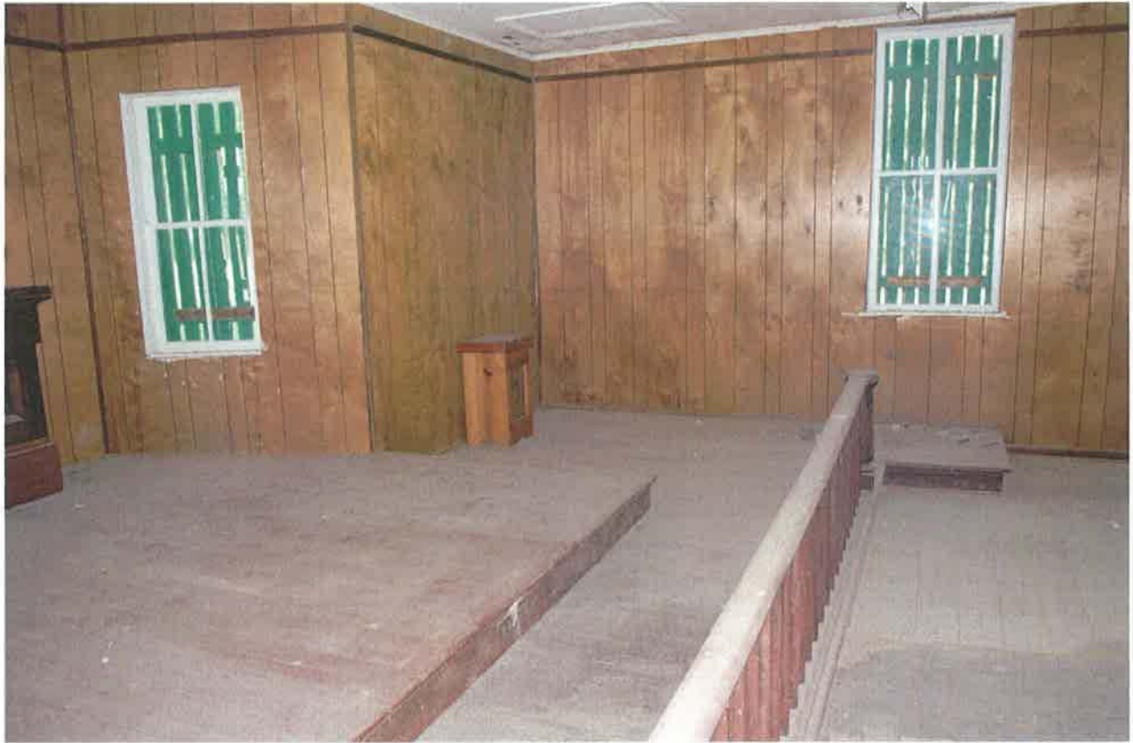
MD_DorchesterCounty_HughesAMEChapel_0005 Interior, facing east
