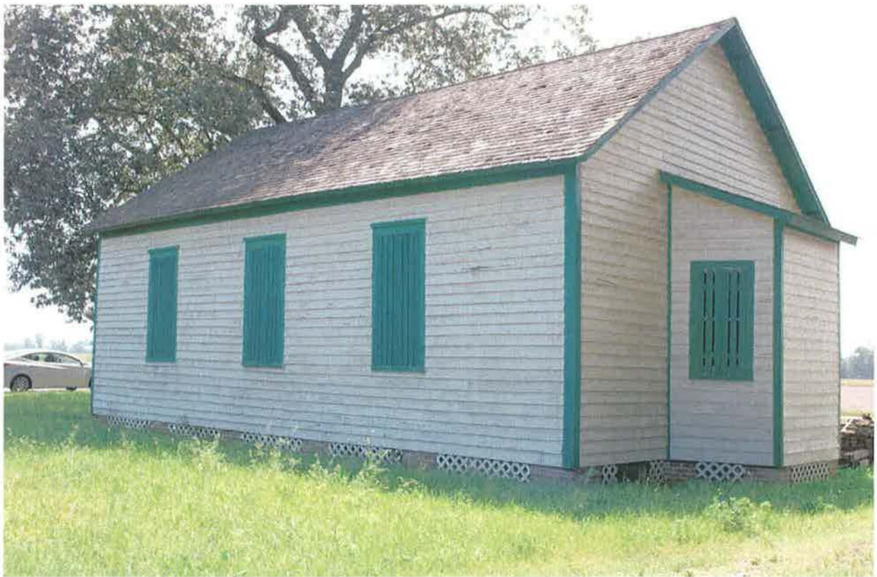
MD_DorchesterCounty_HughesAMEChapel_0002 Exterior, view from northeast
