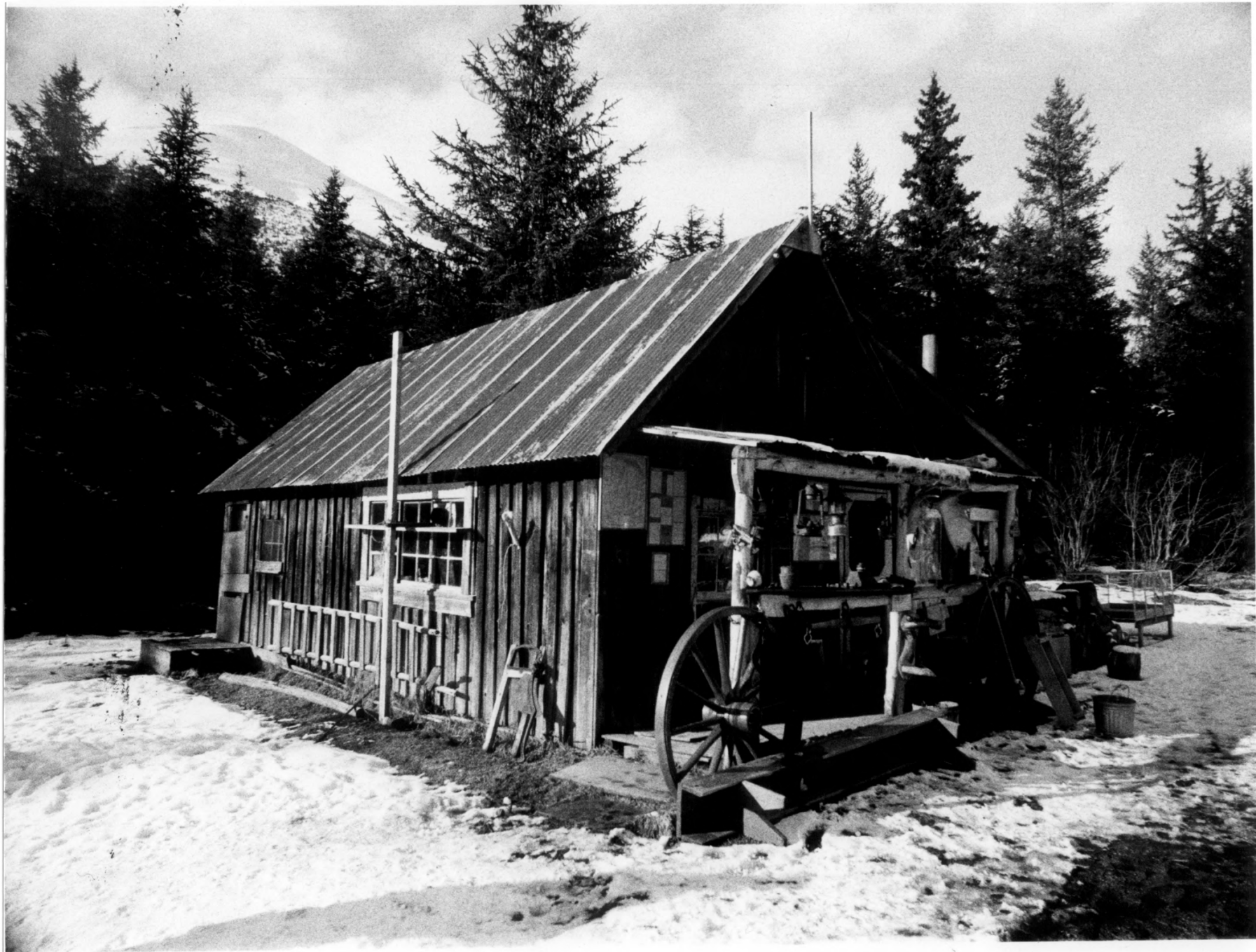
MESS HALL, CROW CREEK MINE
