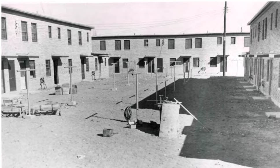
Figure 8 – 1952 View of the rear laundry yards of Apartment Building Type A and Type E taken during construction. Courtesy of the Housing Authority of El Paso archives. See Photograph 3 for a current view of the same location.
