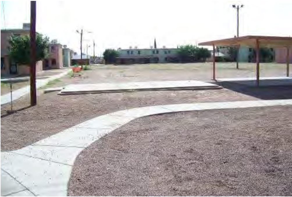
Photograph 21 – Open recreation area and non-contributing metal pavilions and laundry slabs. Camera facing east. (Sept. 2, 2015)
