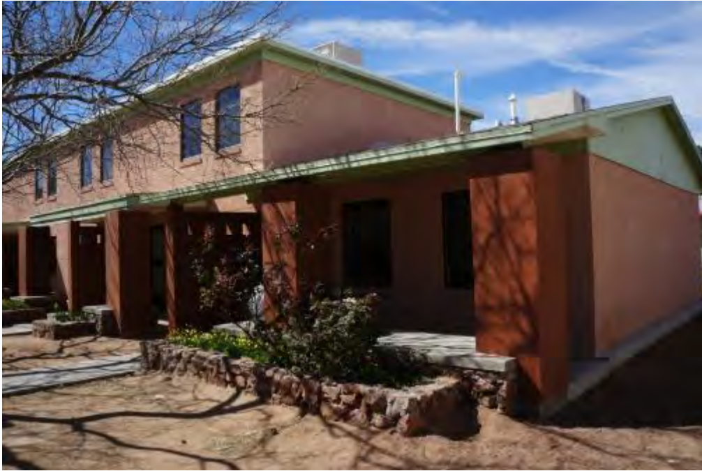
Photograph 3 – Entry Elevation of Apartment Building Type A – porch detail. Camera facing northeast. (March 1, 2016)
