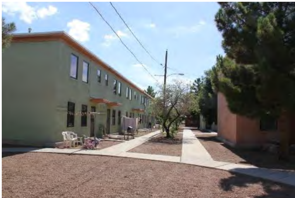
Photograph 7 –Rear façade for Apartment Type C (left) faces the end façade and rear yards of Apartment Type B (right). Camera facing west. (June 28, 2016)
