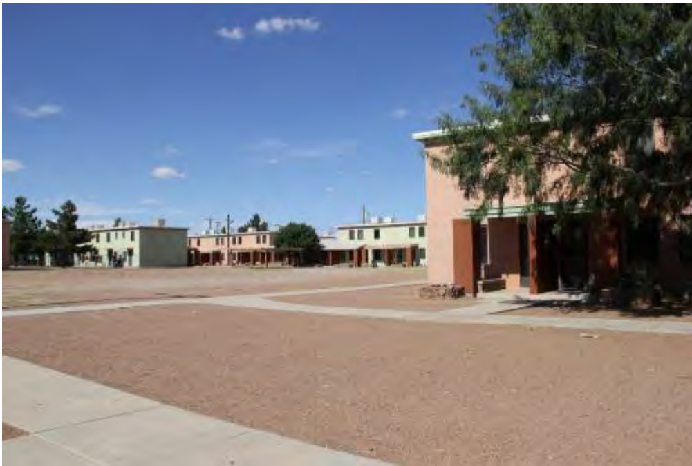
Photograph 4 – View of recreation area and non-contributing metal pavilion, with superbloc of Ray Sherman Place with Apartment Building Type B (right) and Type E (far left) and Type A (center). Camera facing northeast. (June 28, 2016)
