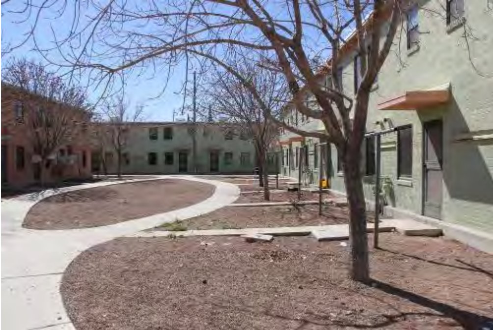
Photograph 1 – View of the rear laundry yards of Apartment Building Type A and Type E. Camera facing north. (March 1, 2016)
