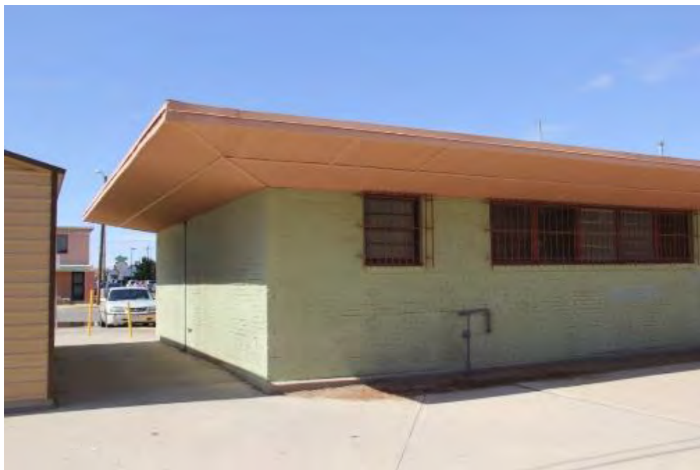
Photograph 17 – Maintenance Building view of west façade (left) and south façade (right). Camera facing northeast. (June 28, 2016)
