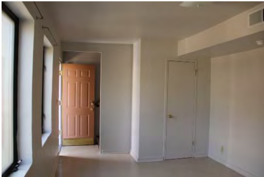
Photograph 19 – Interior view of typical first floor at the entry door area in Apartment Type E. (March 1, 2016)
