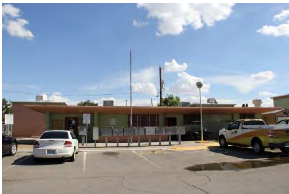
Photograph 14 – Maintenance Building north entry façade along Blanco Avenue. Camera facing south. (June 28, 2016)
