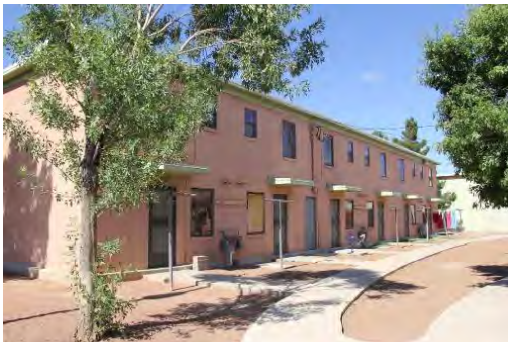
Photograph 13 – Rear façade for Apartment Type E. Camera facing east. (June 28, 2016)
