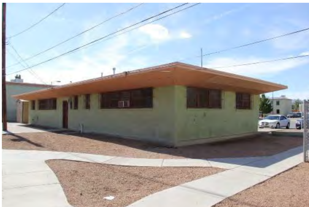
Photograph 16 – Maintenance Building view of south façade (left) and east façade (right). Camera facing northwest. (June 28, 2016)
