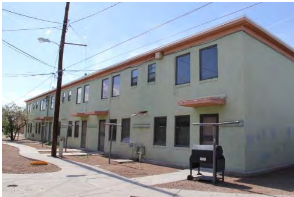
Photograph 11 – Rear façade for Apartment Type D. Camera facing west. (June 28, 2016)
