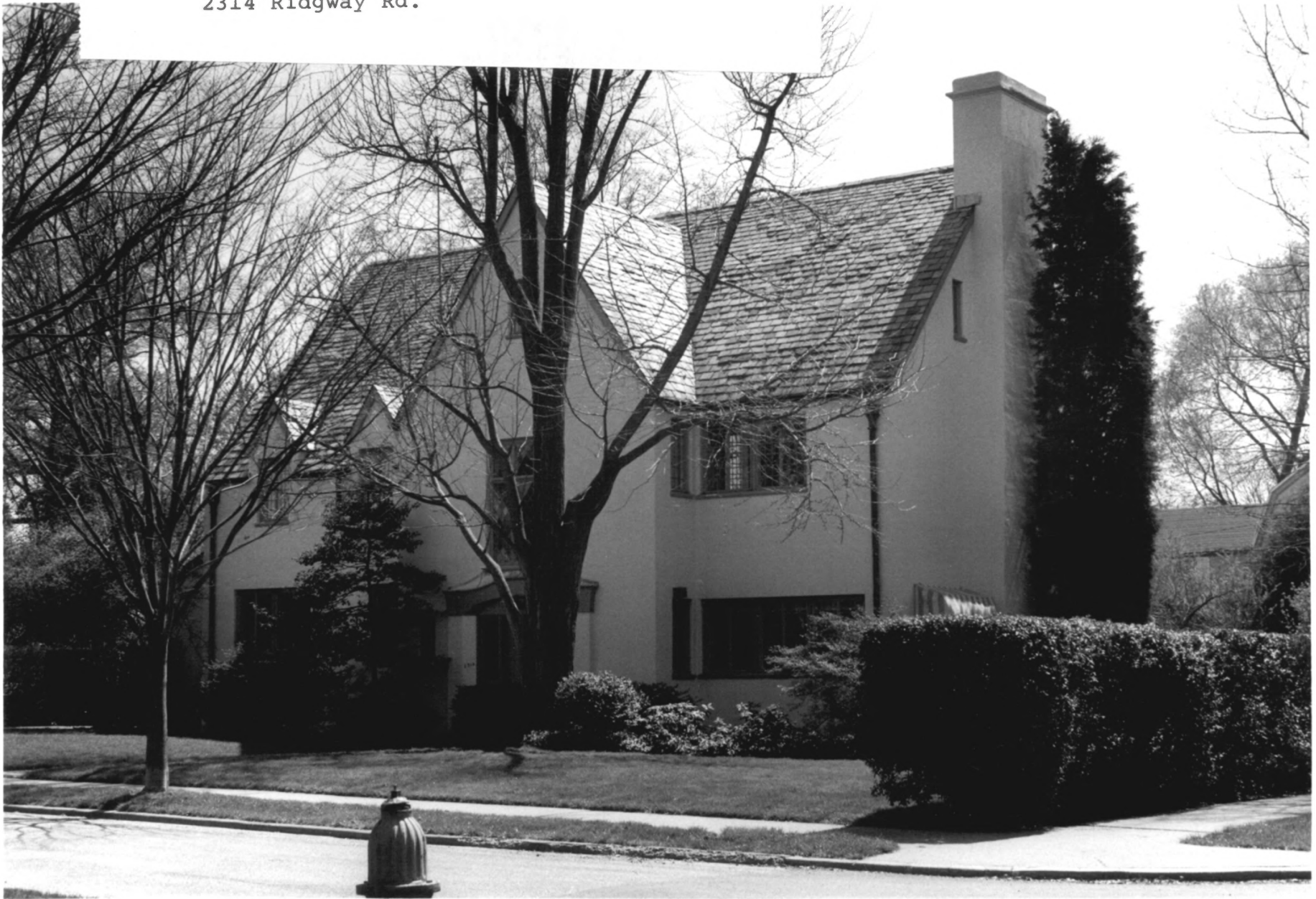
Wawaset Park Historic District Photo #15 2314 Ridgway Rd.
