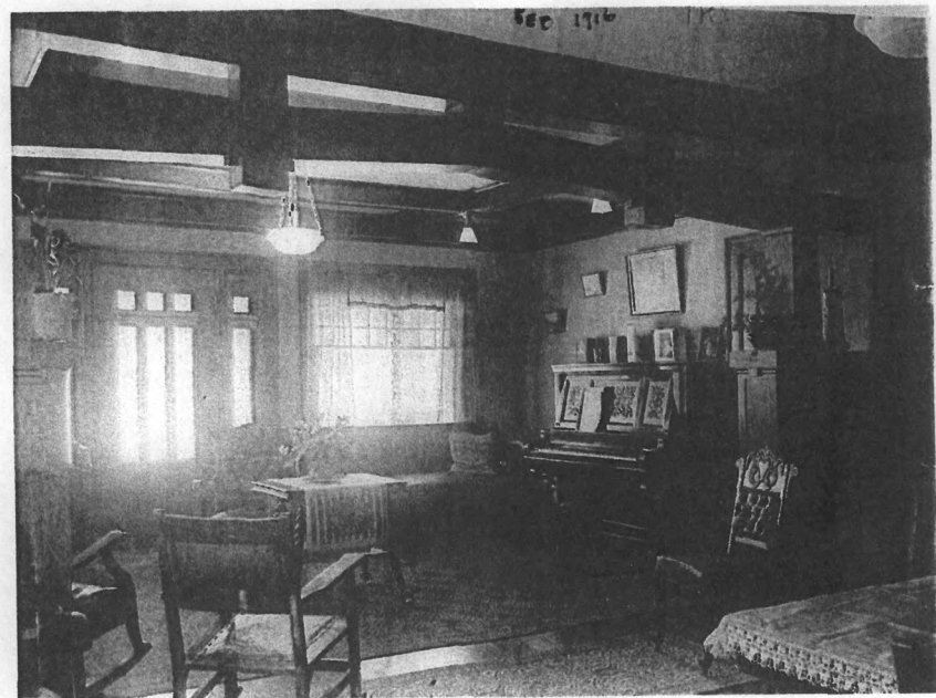
904 Highland Ave. - views of Living Room
