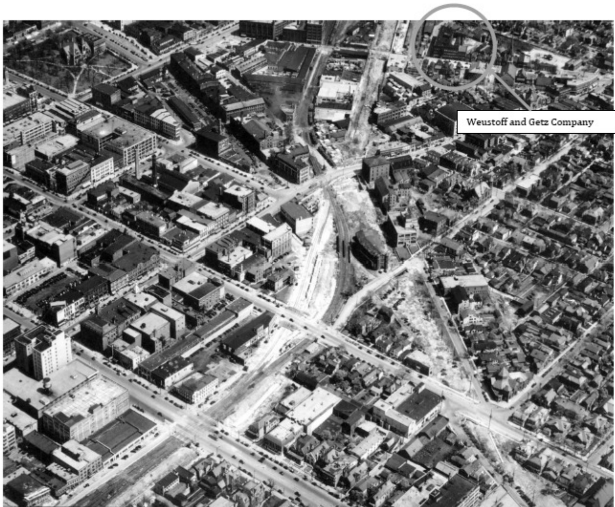
Figure 12: Aerial Photograph of Dayton, ca. 1930, showing the filling of the canal and elevated railroad, with the Weustoff and Getz Company building identified (Source: City of Dayton).
