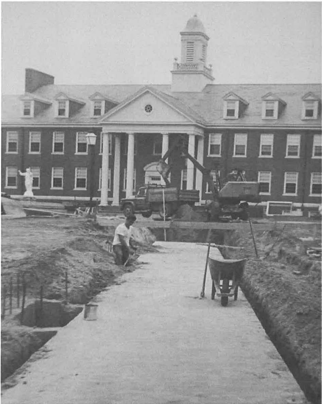
Figure 8: The Construction of the Tunnel, 1959 (courtesy of the Cushing Center Archives)
