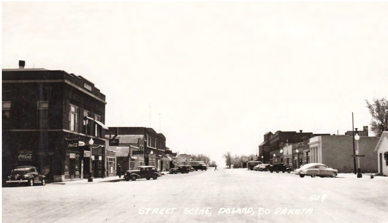
Fig 3 - View of Humphrey Drive, facing south. Buildings on the right are still extant and part of the Doland Historic Commercial District. Buildings on the left, except for the Riley Block in the foreground, have been demolished. Photo c. 1940s.
