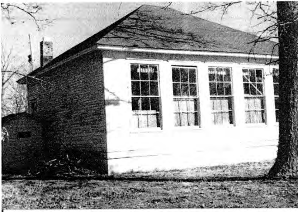
Figure 8, left: the rear (west) and north side elevation, ca. 1985. [Estell Manor Historical Society]
