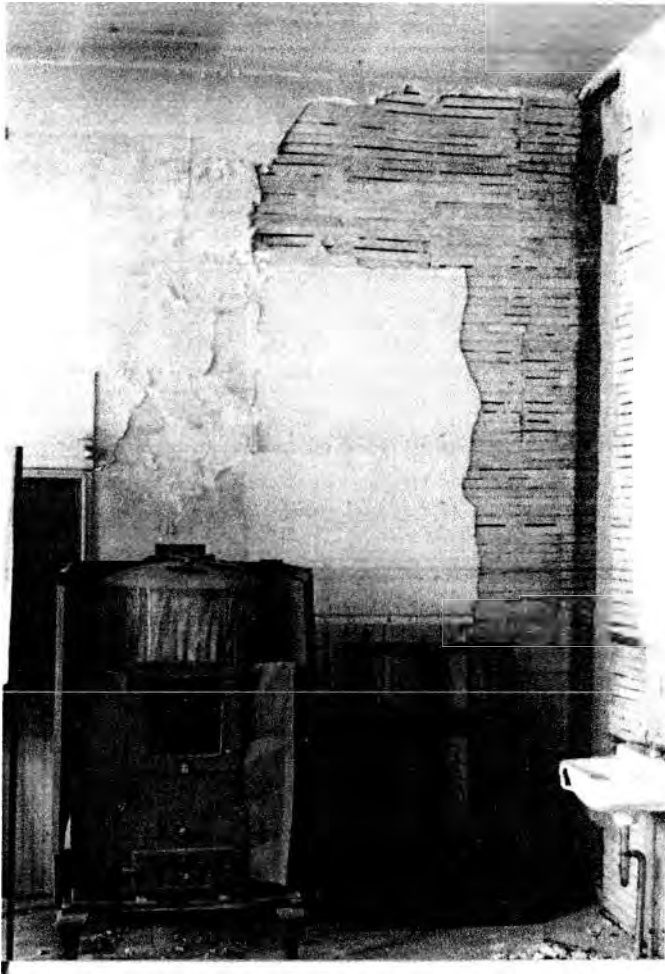
Figure 5, left: the northeast corner of the classroom, looking north, ca. 1985. The heating stove seen here (no longer extant) was vented into the chimney in this corner and the stovepipe opening is visible near the ceiling. Note the water fountain nearby. This corner of the classroom is now enclosed and contains the modern HVAC equipment. [Estell Manor Historical Society]
