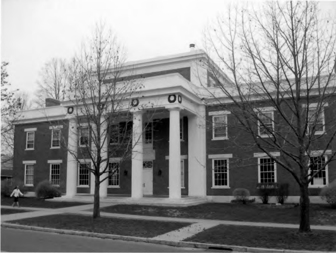
Photograph 0001: Eclectic Society House, Middletown, CT Exterior view of the west elevation; camera facing northeast
