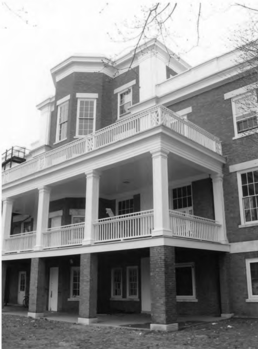
Photograph 0005: Eclectic Society House, Middletown, CT Exterior view of the east and north elevations; camera facing southwest
