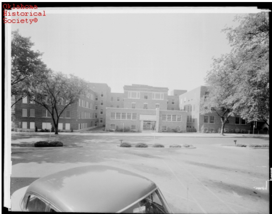
FIGURE 7: Wesley Hospital circa 1953, showing entrance addition. This is how the nominated building appears today. (Source: Oklahoma Historic Society)
