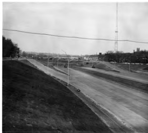
Figure 9: Interstate 480 at its near completion. The non-contributing television tower within the district boundaries is visible at the right side of image. Photo taken November 15, 1962 and courtesy of the Robert Paskach Collection of the Durham Museum.
