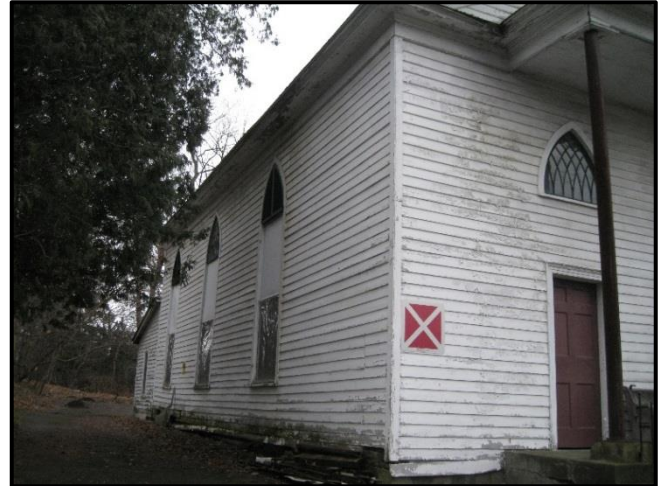
Figure 15. East elevation (January, 2017). Note window construction.
