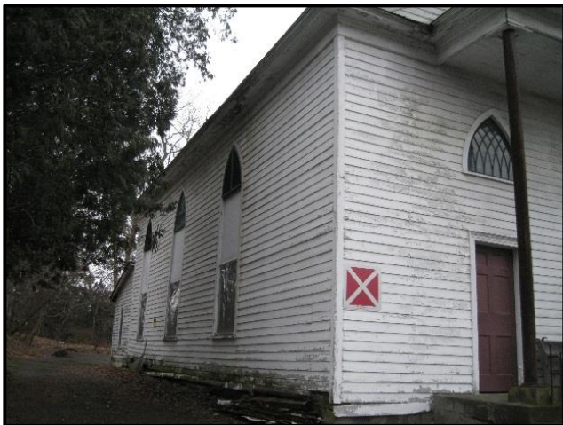
Figure 4. Side (east) elevation, 2017.
