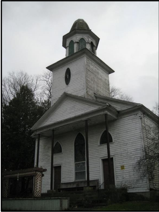
Figure 14. Façade (north) (January, 2017). Elements of the steeple and lantern resemble those of other early nineteenth century meeting houses.
