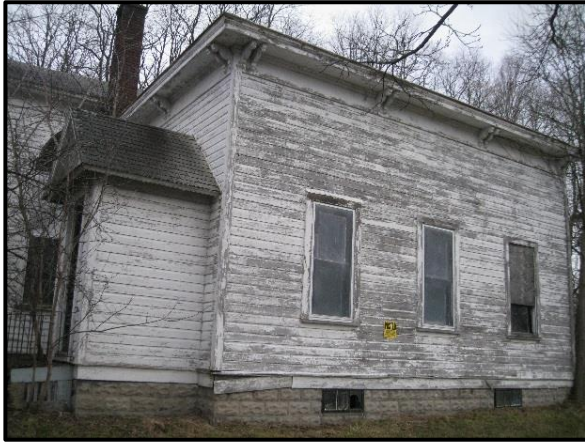
Figure 6. Side (west) elevation of session room, 2017.
