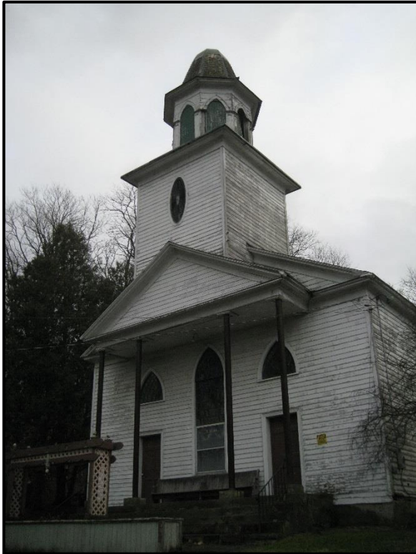
Figure 2. Wampsville Presbyterian Church, façade, 2017.
