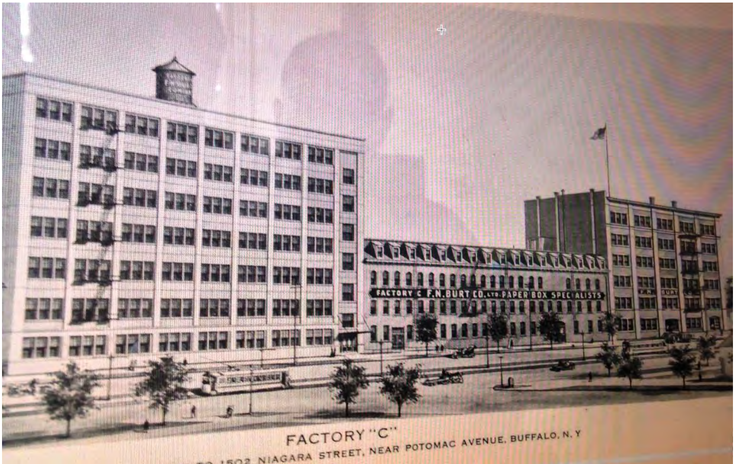
Figure 1. Rendering of Factory "C" (ca. 1920). Seven-story reinforced concrete factory building next to four-story and six-story buildings formerly Baynes Carriage Works. Source "Big Deal: 1502 Niagara Street Purchased," Source: Buffalo Rising Online . Refer to Figure 8 showing the buildings on the 1916 Sanborn Map.
