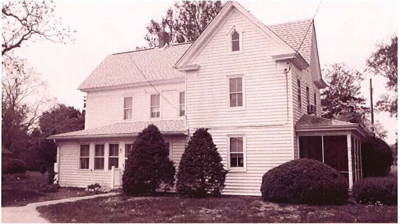
D.E. Sussex County Stone-Well House Northeast three-quarter elevation
