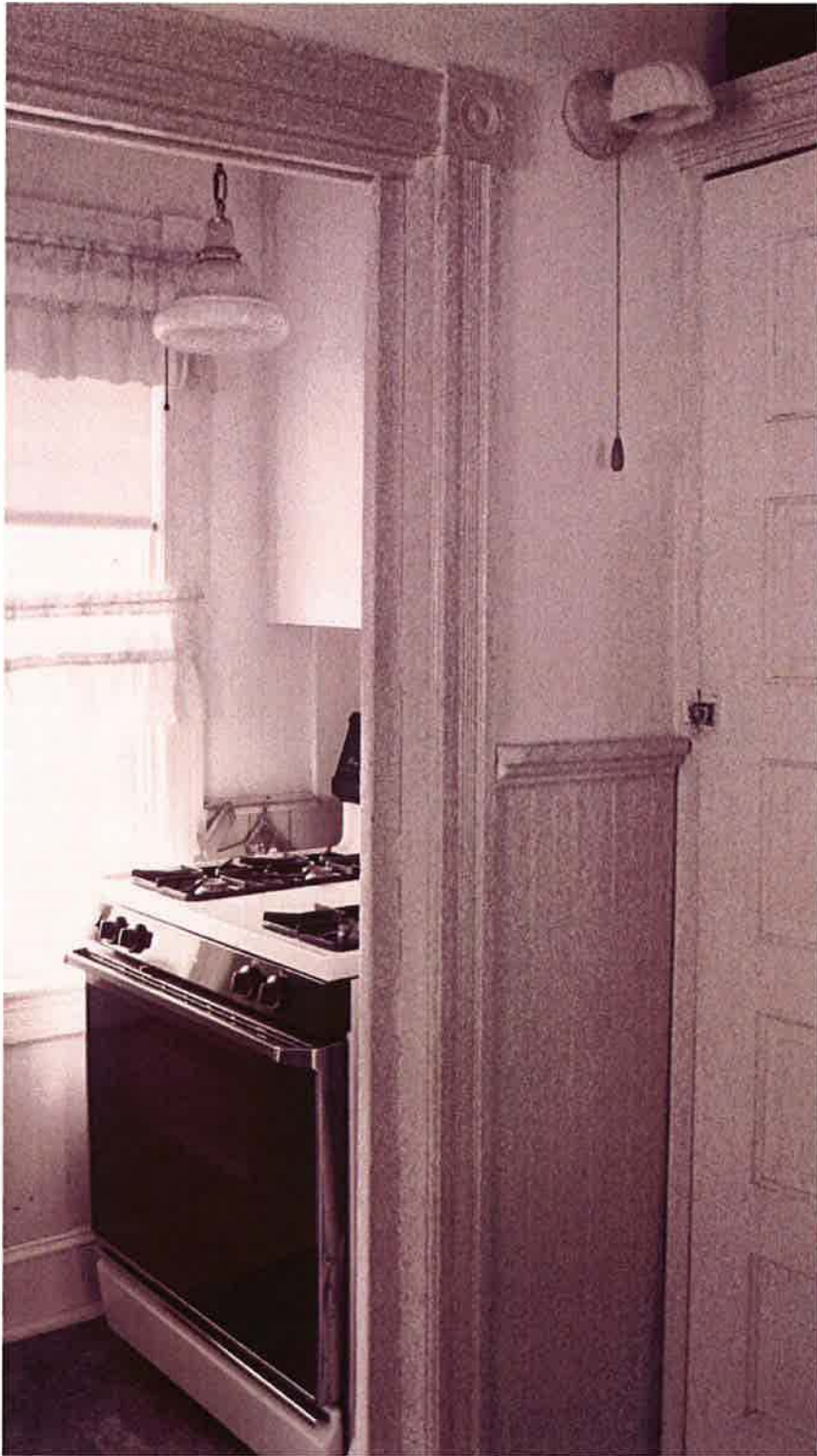
03 Sussex County, Evans-Weat House West kitchen area with original wainscoting and molded door surrounds with bull-eye corner block trim
