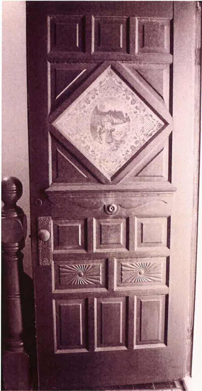
DB Sussex County Evans-Weat House original exterior door (main facade) with decorative wood panel trim and frosted etched glass window
