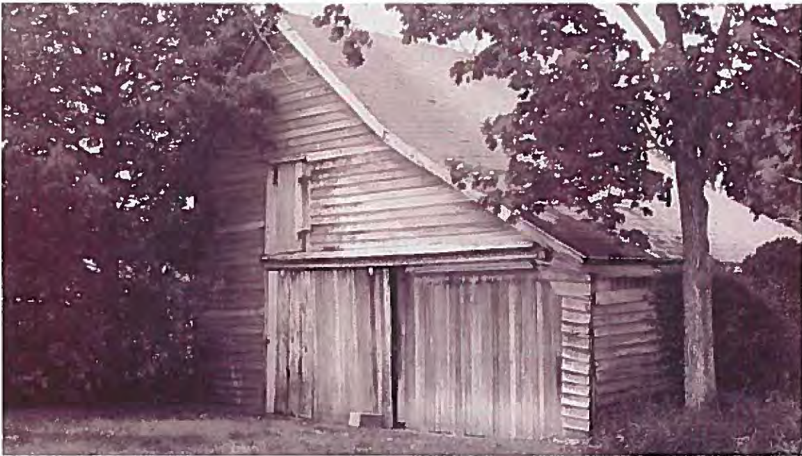
DE Sussex County Evans-West House East elevation of the Evans-West House built approximately 1900 11 of 14
