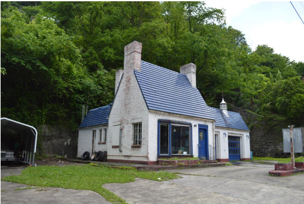
Photo 18: 194 Wyoming Street, Pure Oil/Union 76 Service Station, North and West Elevations, Facing Southeast
