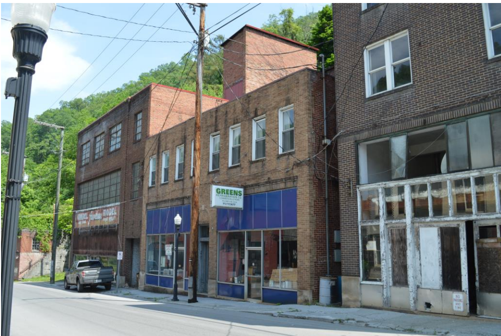
Photo 9: 162 Wyoming Street, Green's Refrigeration Company, façade (West Elevation), Facing Northeast
