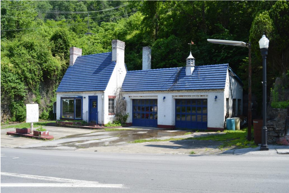
Photo 17: 194 Wyoming Street, Pure Oil/Union 76 Service Station, façade (West Elevation), Facing East
