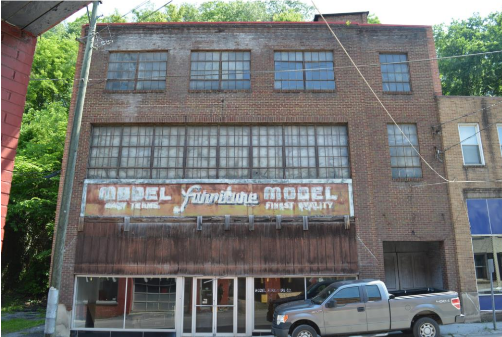
Photo 10: 170 Wyoming Street, Model Furniture Building, façade (West Elevation), Facing East
