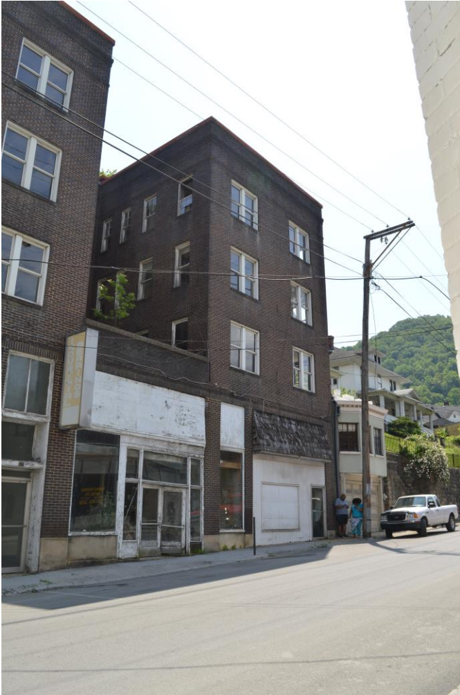
Photo 7: 154 Wyoming Street, Wyoming Court Apartments, Corner of West and North Elevations, Facing Southeast
