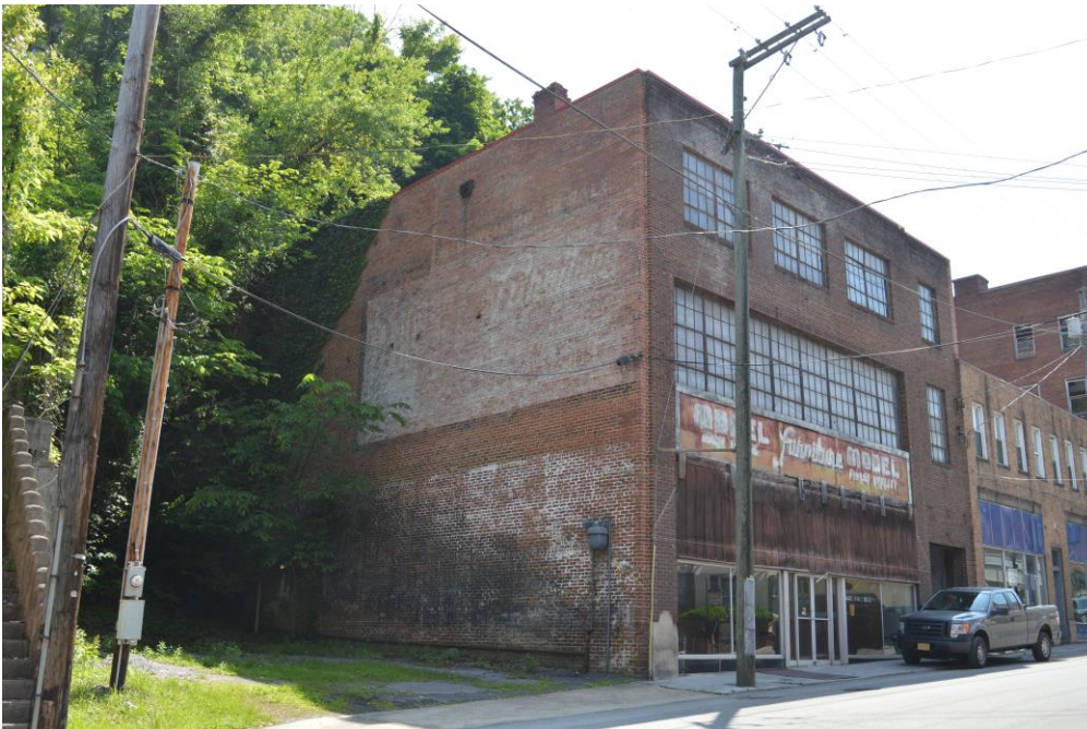
Photo 11: 170 Wyoming Street, Model Furniture Building, North and West Elevations, Facing Southeast
