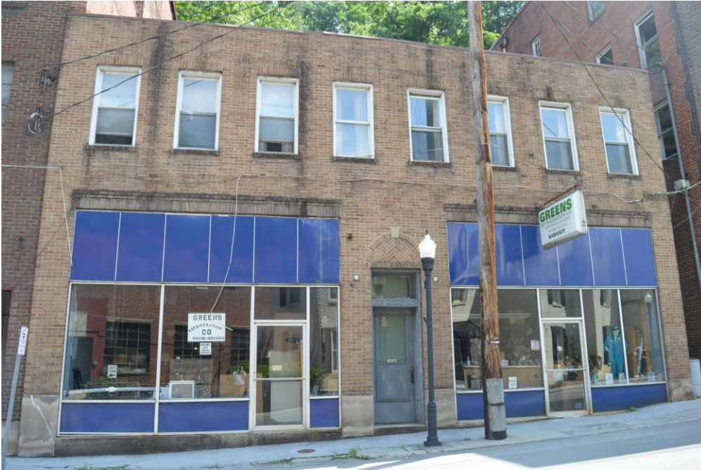
Photo 8: 162 Wyoming Street, Green's Refrigeration Company, façade (West Elevation), Facing East
