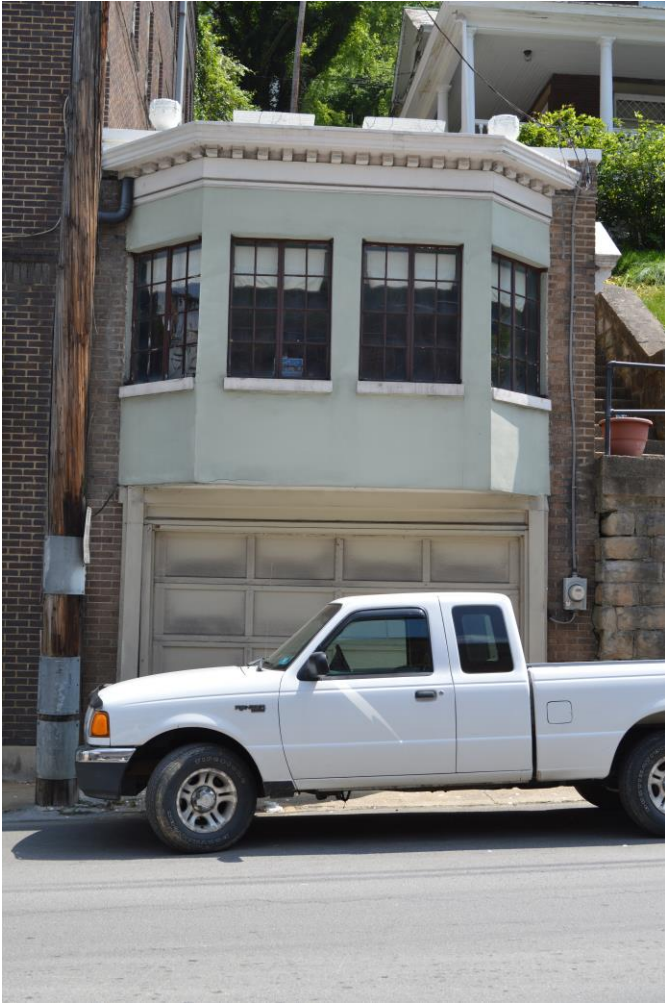
Photo 3: 142 Wyoming Street, Ashworth House Garage/Apartment, façade (West Elevation), Facing East
