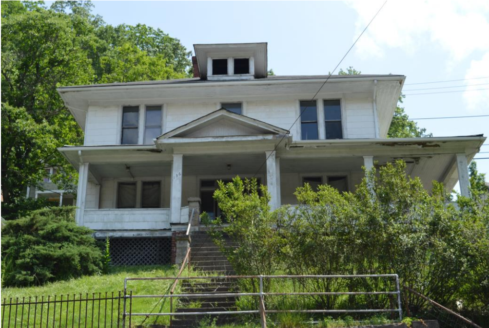
Photo 1: 136 Wyoming St., Facade, Facing east
