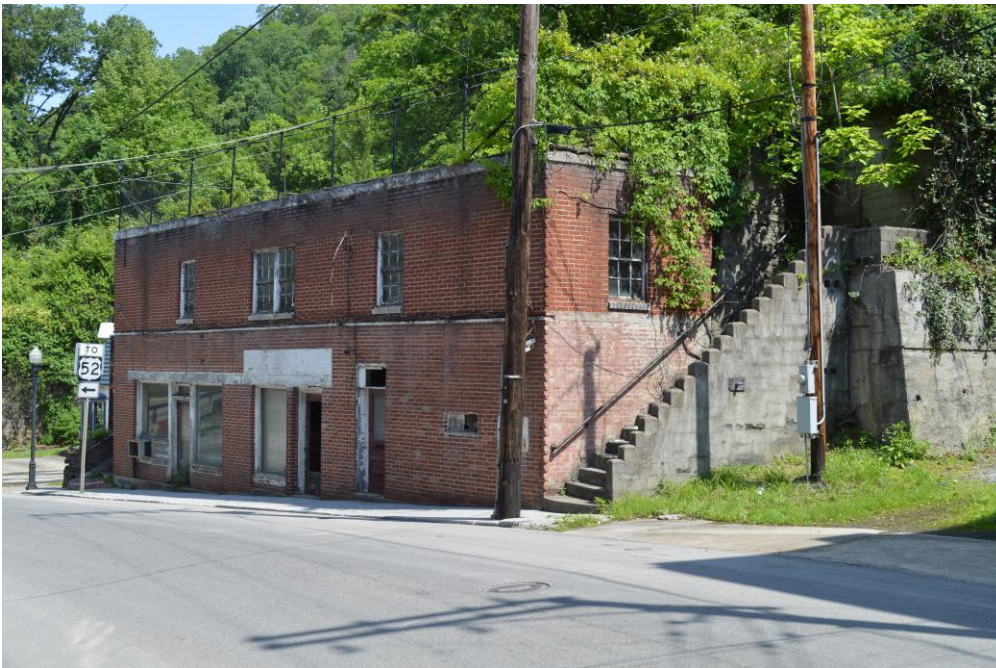
Photo 16: 182 Wyoming Street, Marino Realty Building, West and South Elevations, Facing Northeast
