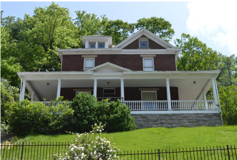
Photo 2: Wyoming St., Facade, Facing East
