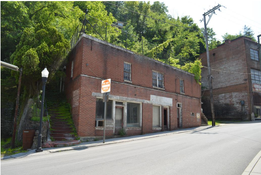
Photo 14: 182 Wyoming Street, Marino Realty Building, North and West Elevations, Facing Southeast
