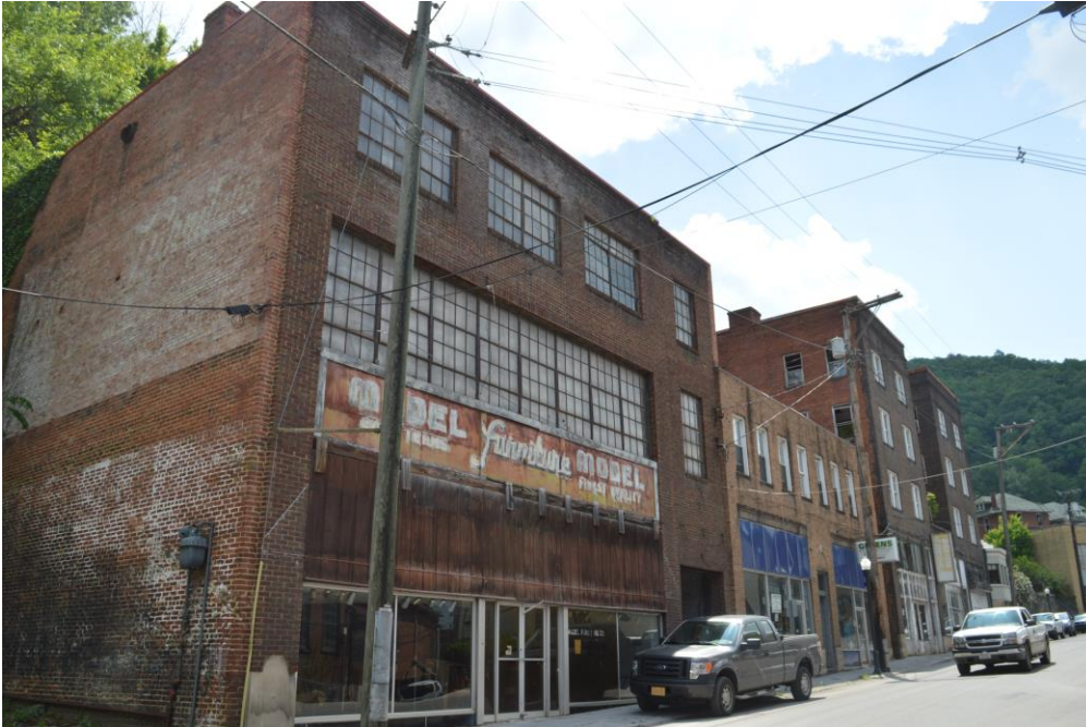
Photo 13: 142, 154-156, 162, & 170 Wyoming Street, Streetscape, Facing Southeast
