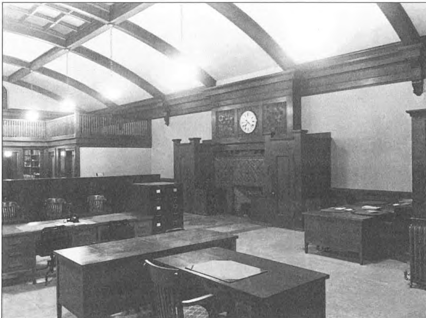
Historic Photograph 3 - Interior looking southeast, c. 1938.
