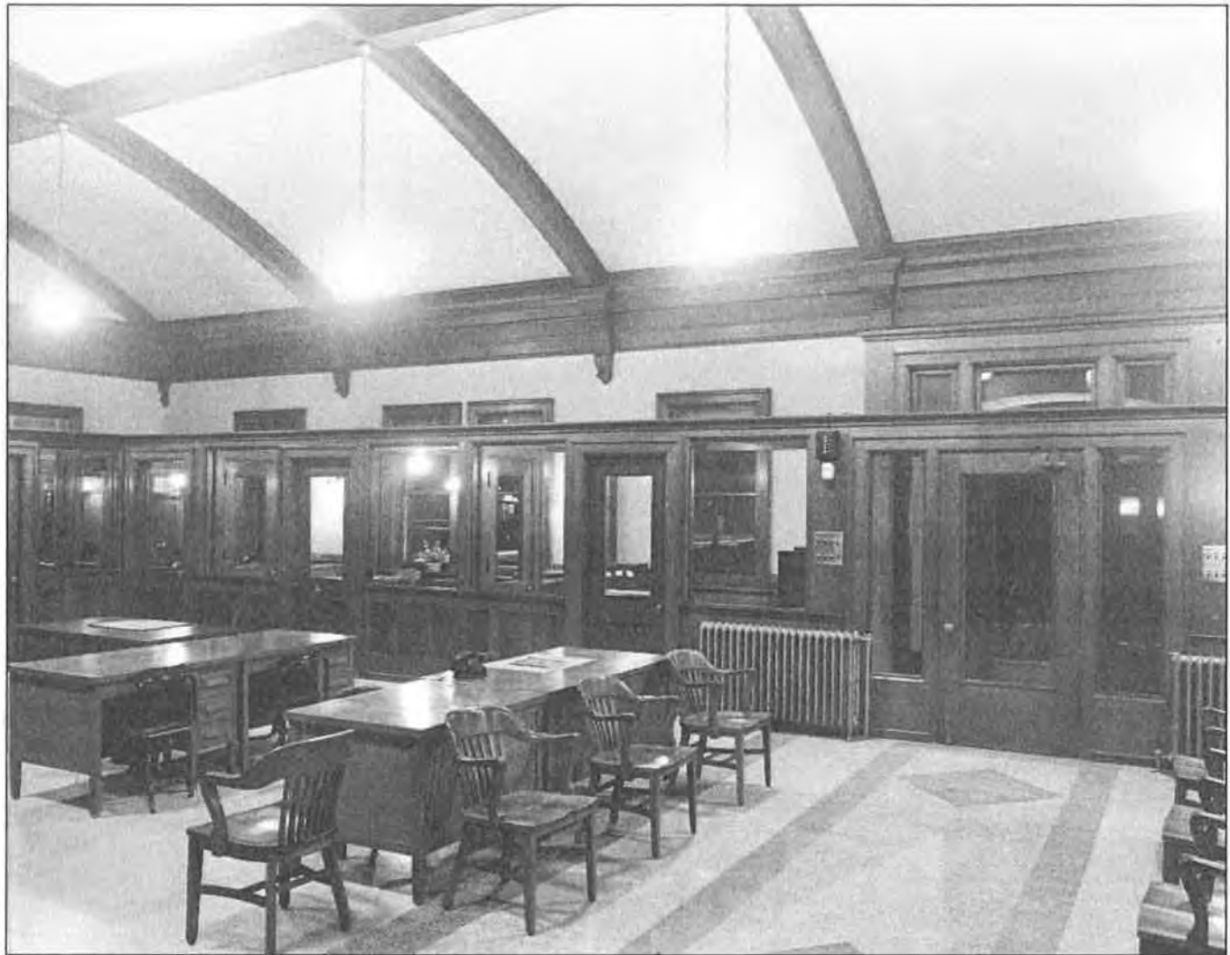
Historic Photograph 2 - Interior looking north to front door, c. 1938.
