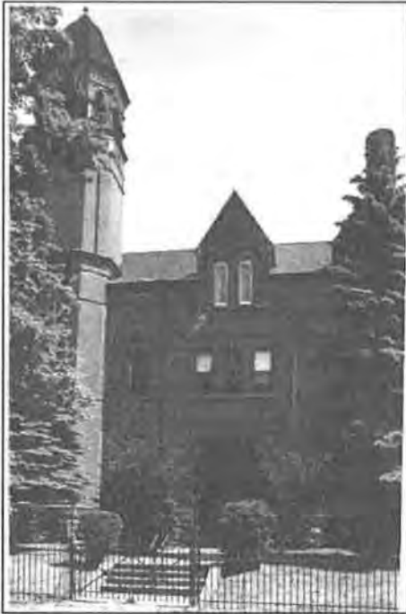
Image 18 - Villa Maria Academy, City of Erie, Erie County, 1892, David K. Dean & Sons, Architects, PHMC CRGIS.
