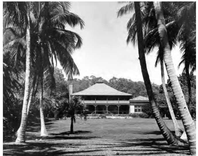
The Barnacle, home of Ralph M. Munroe, and an example of traditional architecture in Coconut Grove.
