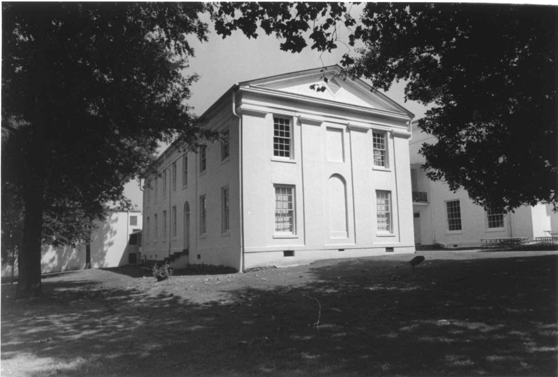
OLD STATE HOUSE Little Rock, Arkansas West temple, south elevation Photo by Mark Christ, 9/96
