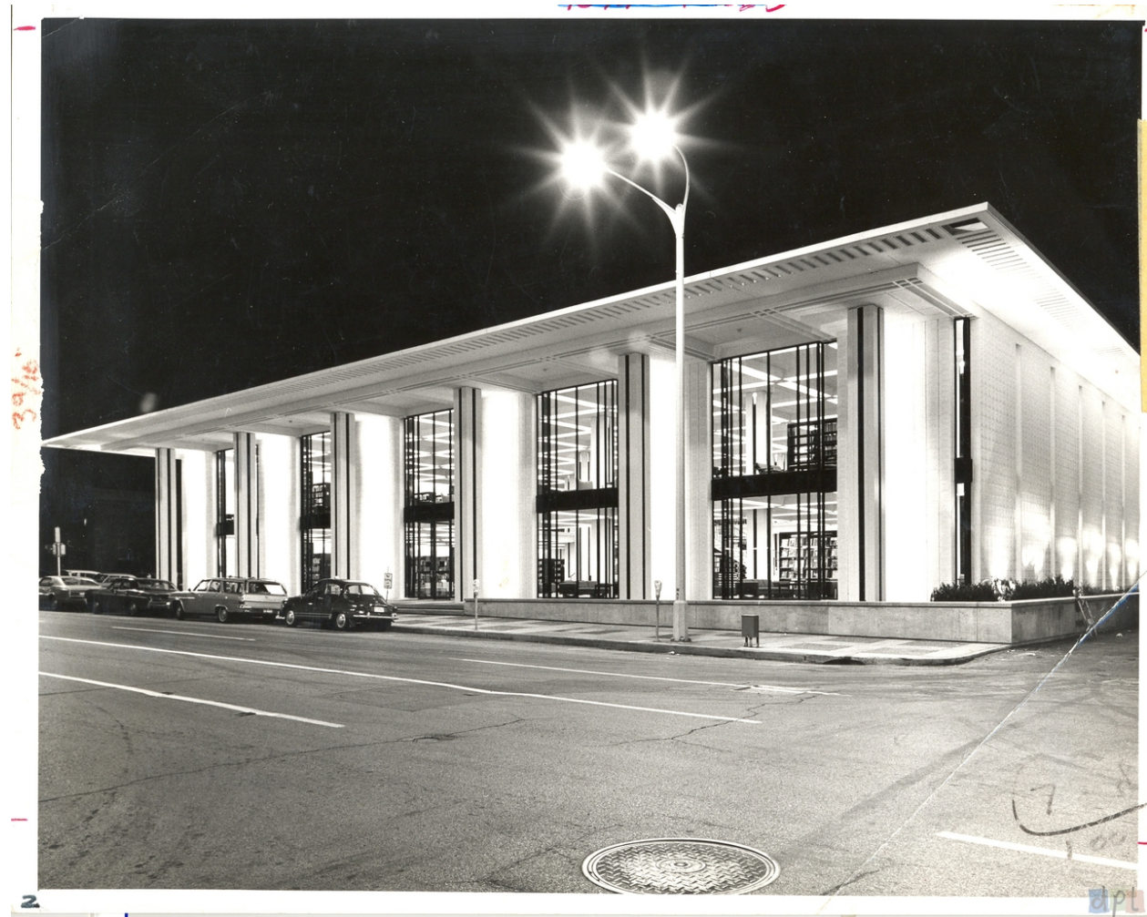
Figure 15: The Davenport Public Library upon completion in 1968. Source: Collection of the Davenport Public Library.
