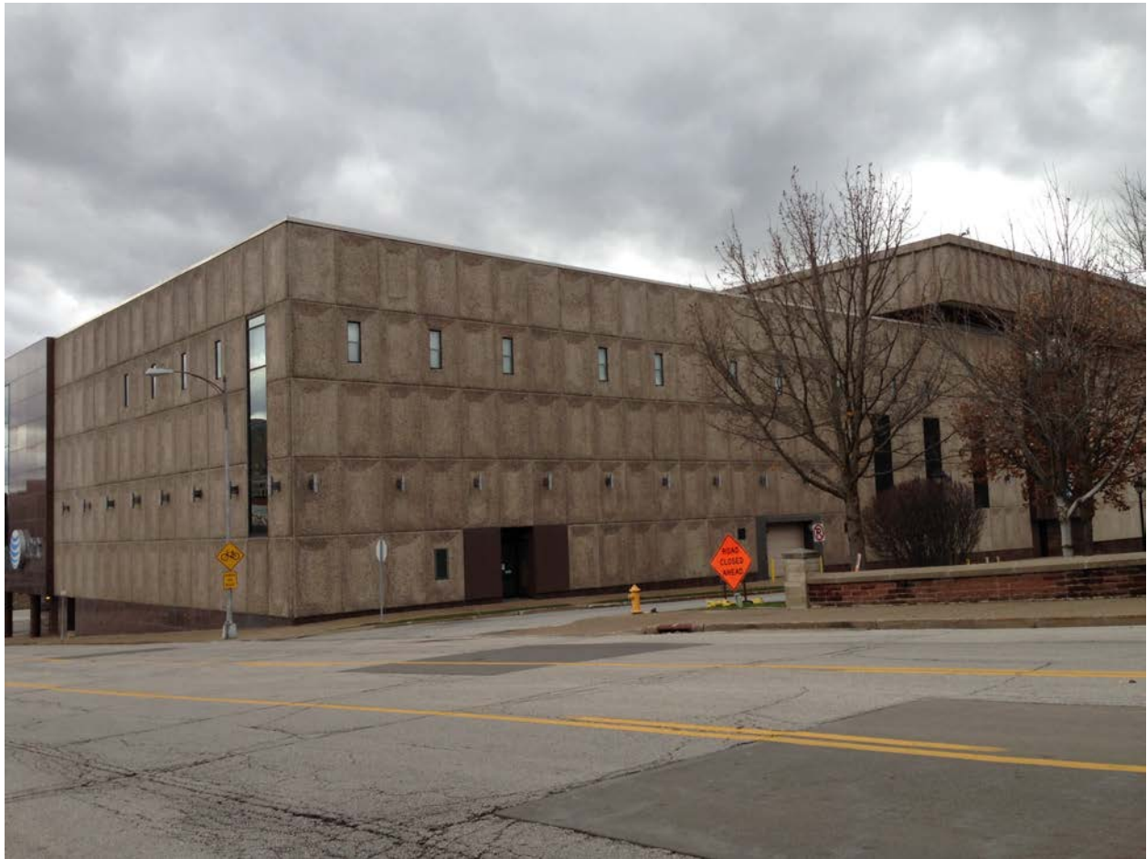
Figure 13: Northwestern Bell Telephone Company Building, re clad in 1965. Source: Photograph by preparer, November 2015.
