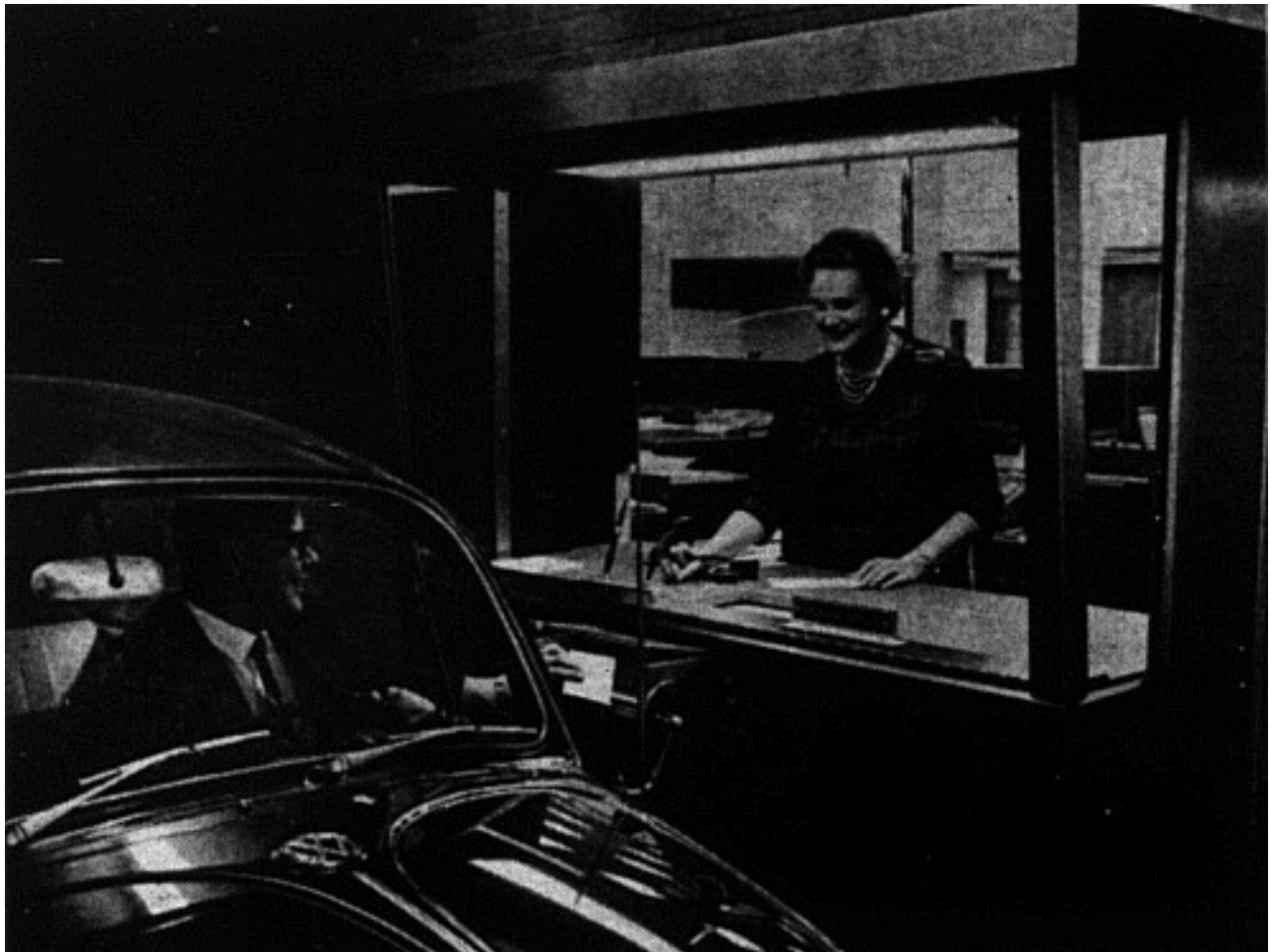
Figure 22: The First Federal Savings and Loan Association Building drive-through with teller window (location still extant, window removed) at its opening in 1966. Source: First Federal Savings Advertising Section, Davenport Times-Democrat , 26 June 1966.
