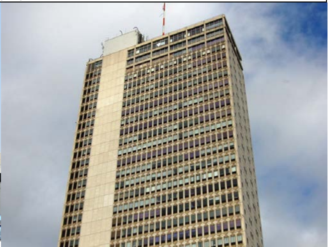
First National Bank of Mobile Building; 1965; Mobile, Alabama. Source: Defining Downtown website, accessed 2016.
