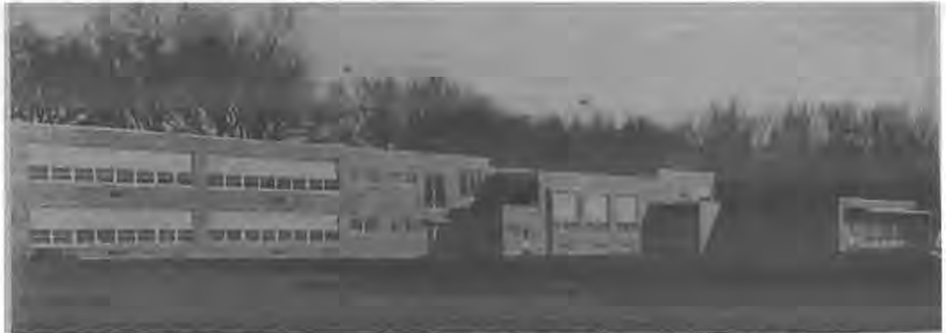
Figure 22 Photograph published in the Clinton Herald on 12/9/1953 of the south elevation of the new Jefferson school (looking northeast). The 1934 building is off the left side of this view but not visible. Today, a modern modular classroom sits in front of roughly the central portion of this photo.
