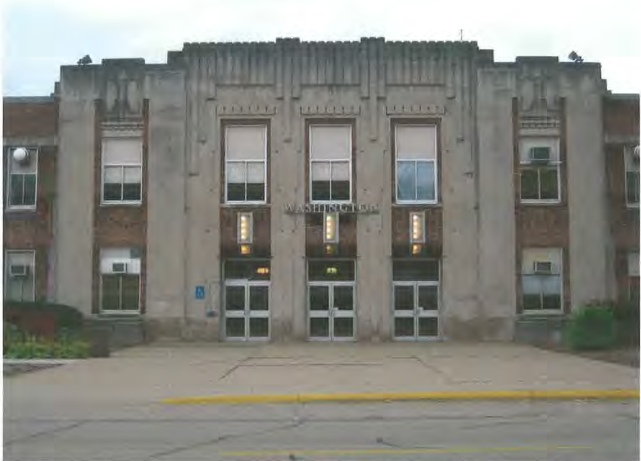
Figure 2 Doors of the central entrance pavilion are framed in white metal, as is the name “Washington” overhead. Tallgrass Historians L.C., 2014
