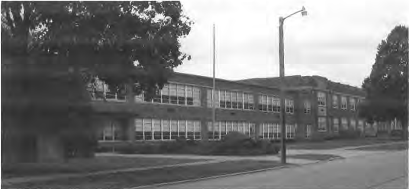
Figure 5 The main entrance to the addition is partially visible behind the bushes on the left. Windows to its right reflect three interior classrooms. Two more such classroom expanses are located to the left of the front entrance and not seen in this view. Tallgrass Historians L.C., 2014
