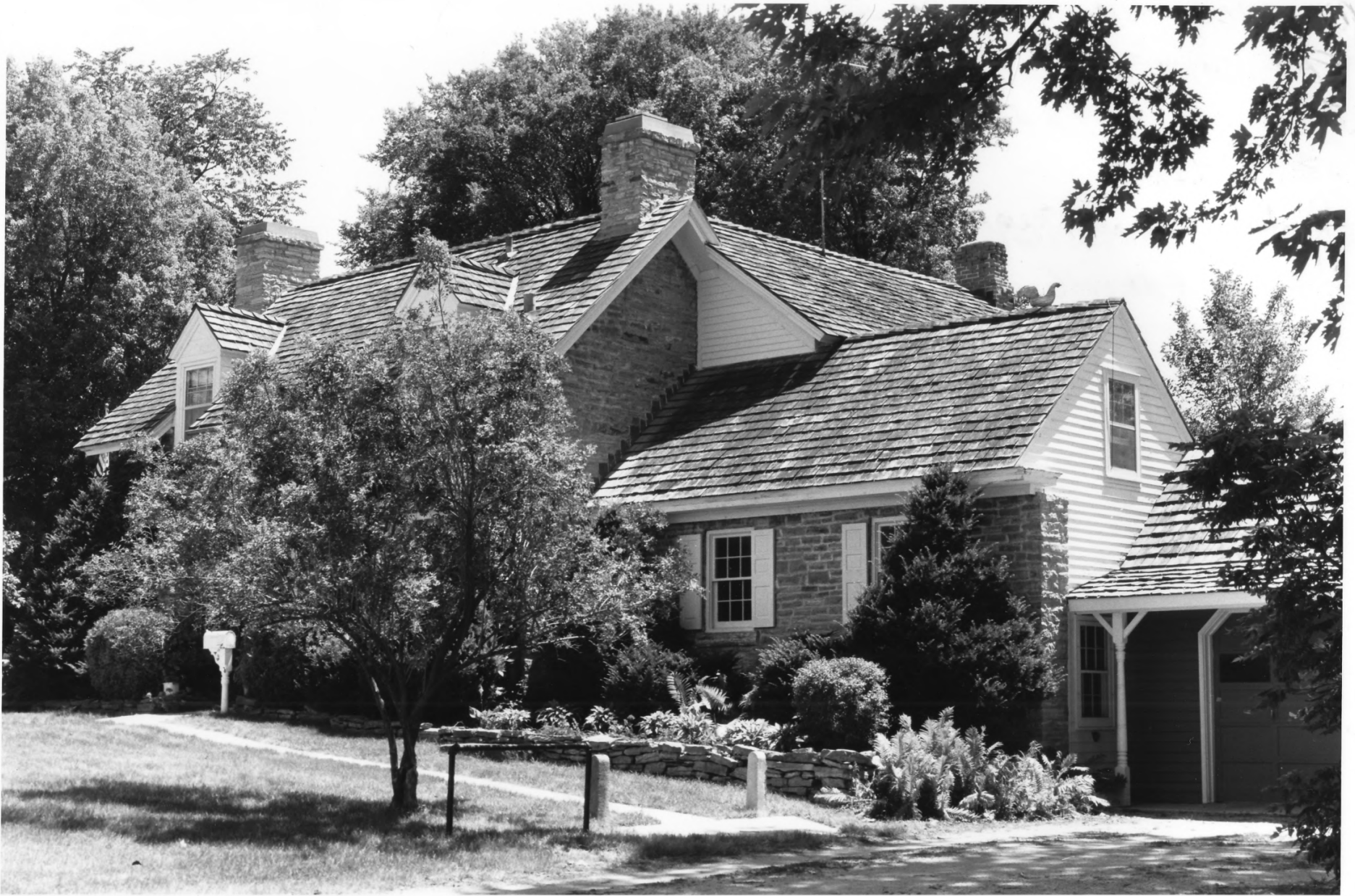
MC CALL, CORMACK, HOUSE FARIBAULT RICE CO., MN PHOTO I. D. 09929 # 3A
