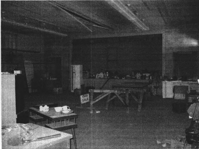
View of the auditorium towards the stage.
