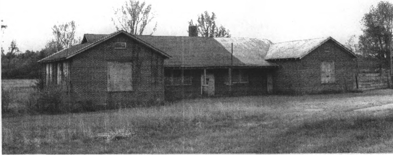
North façade of the Pocahontas School
