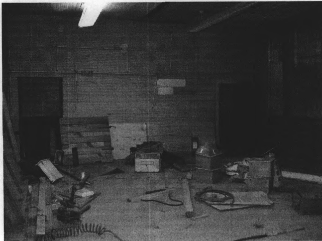
Northeast classroom, view to north.
