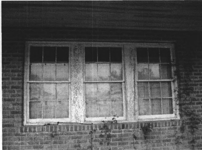
Original windows on the main façade.
