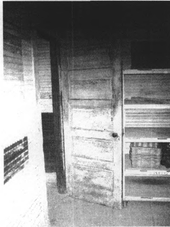
Original five-panel interior door.
