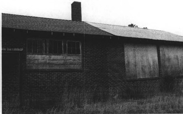
West façade, showing cafeteria and kitchen wings.
