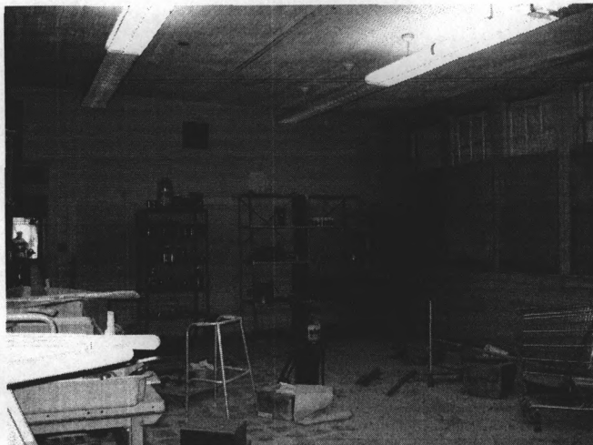
Northwest classroom, view to south.
