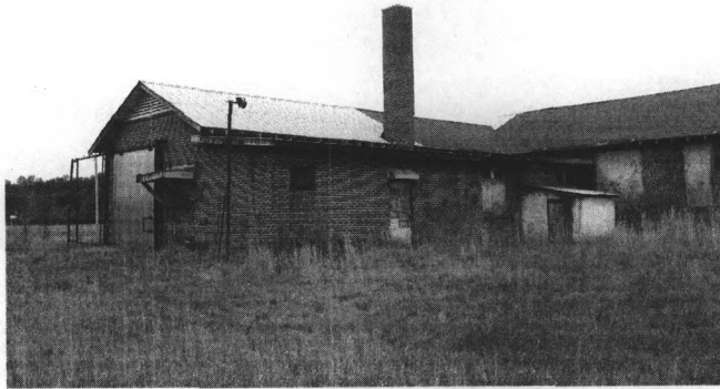
View of the east façade of the 1957 wing, view to northwest.
