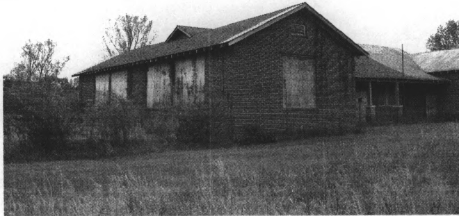
East wing of the school, view to the southwest.
