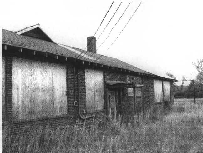
West façade of the west wing.
