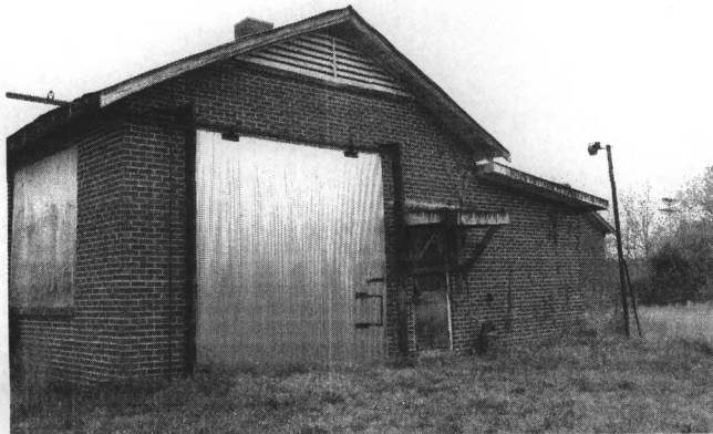
Rear or south façade showing the ca. 1970 added door.
