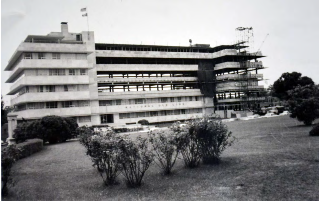
Fig. 8 – National Old Line Building near completion of the addition, ca. 1965
