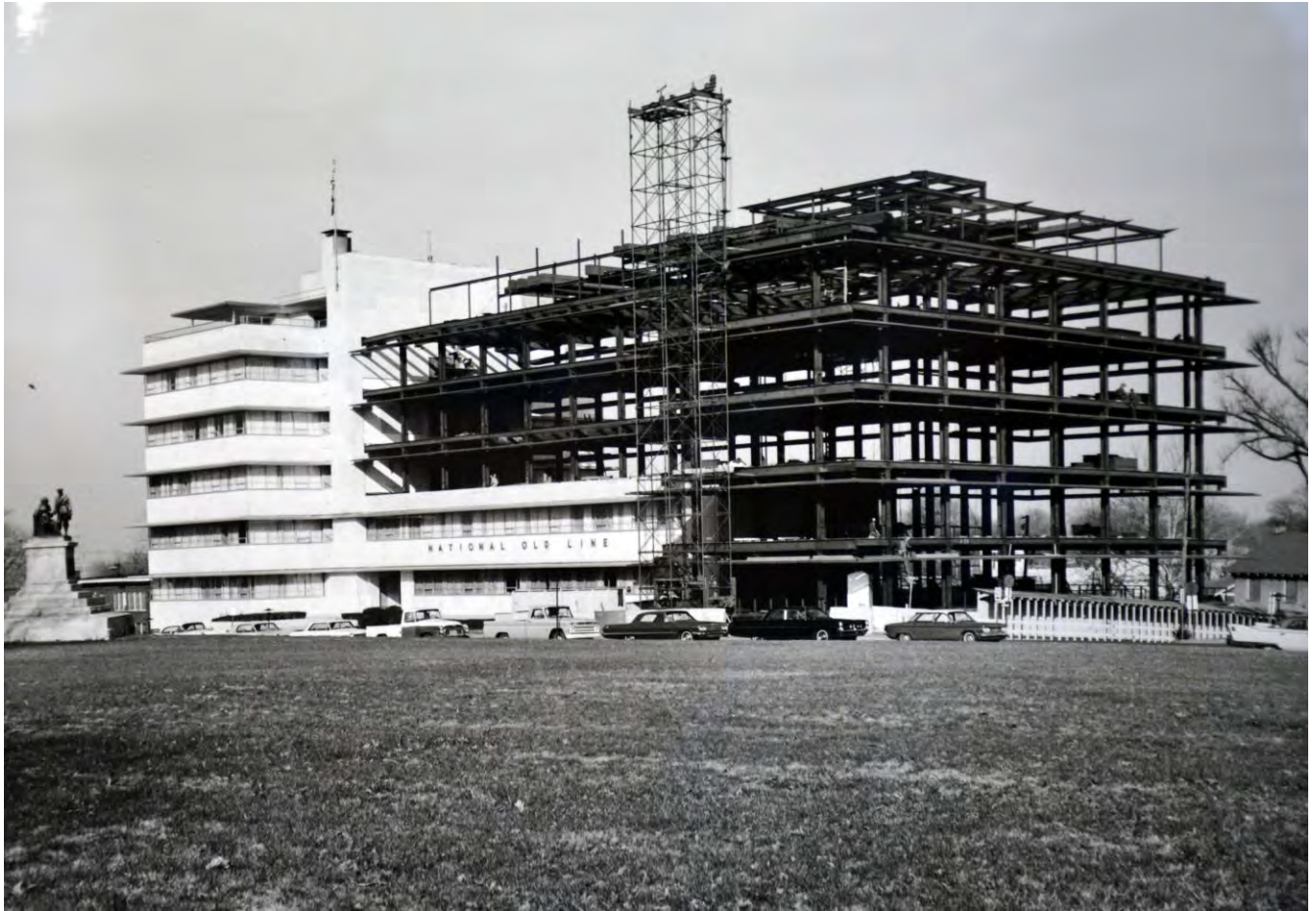
Fig. 7 – National Old Line Building during construction of addition, ca. 1964
