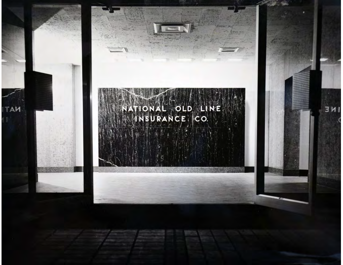
Fig. 4 – Original west entrance
