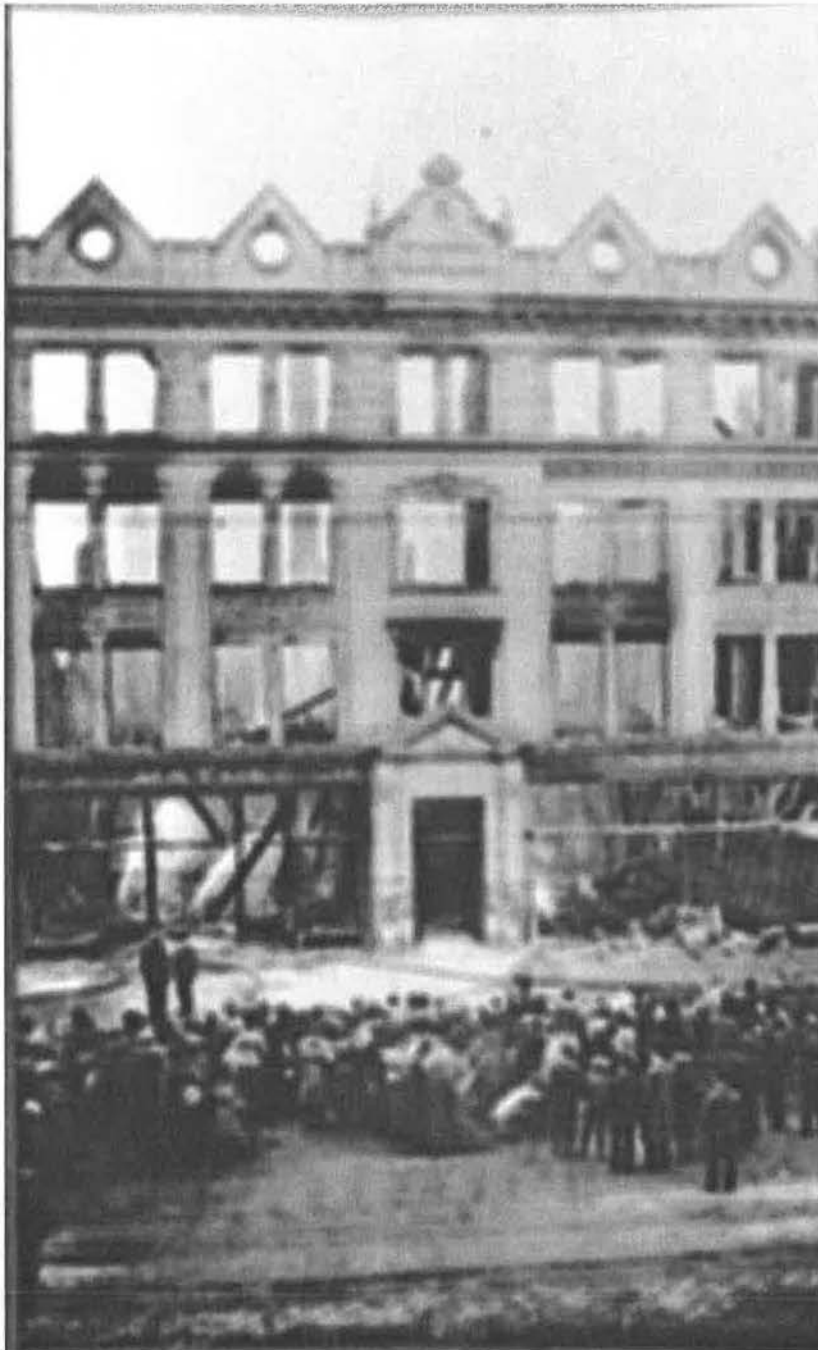
Figure 3: Ruins of the Mehrum Block after the fire, November 1906, Butler County Historical Society
