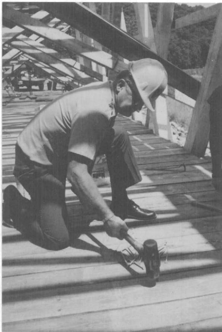
Figure 41: Assistant Superintendent, Operations, Einar L. Johnson drives a nail into the reconstructed Everett Road Covered Bridge, a project undertaken by the National Park Service's Williamsport Preservation Training Center.
